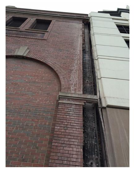
Masonry Removed to Inspect Structural Steel (State St. Substation)
