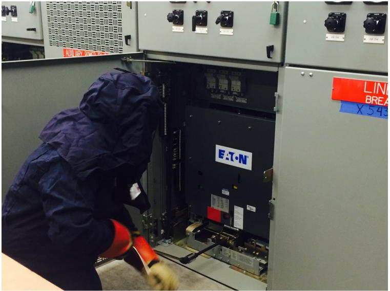
Armitage Substation: Removing Switchgear with PPE
