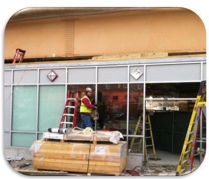
Station House curtain wall, glass, & exterior station electrical fixtures being installed.
