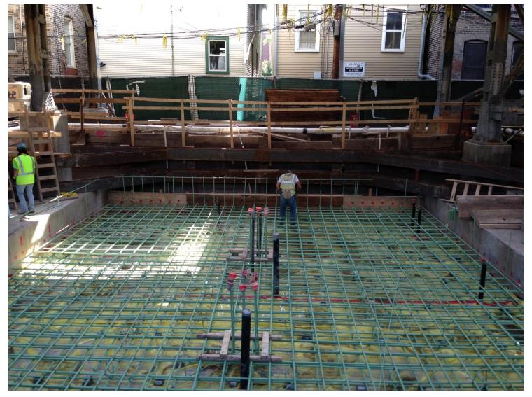
**Armitage Substation: building foundation rebar installation**
