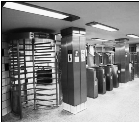
Harrison Station Fare Area After
