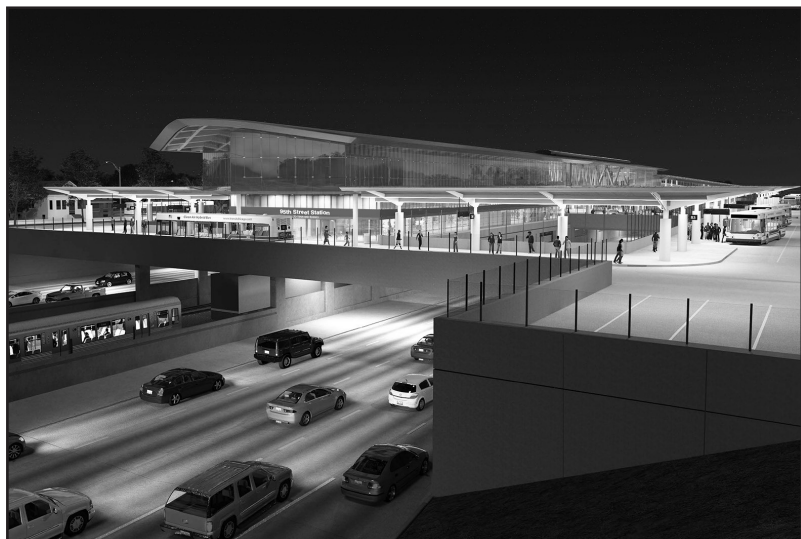
Mayor Rahm Emanuel and elected officials broke ground in September 2014 on the historic $240 million project to reconstruct the 95th Street Red Line Terminal—the city's busiest multi-modal facility. The new, modern and more spacious terminal will be a showcase destination befitting 21st Century transit riders.
