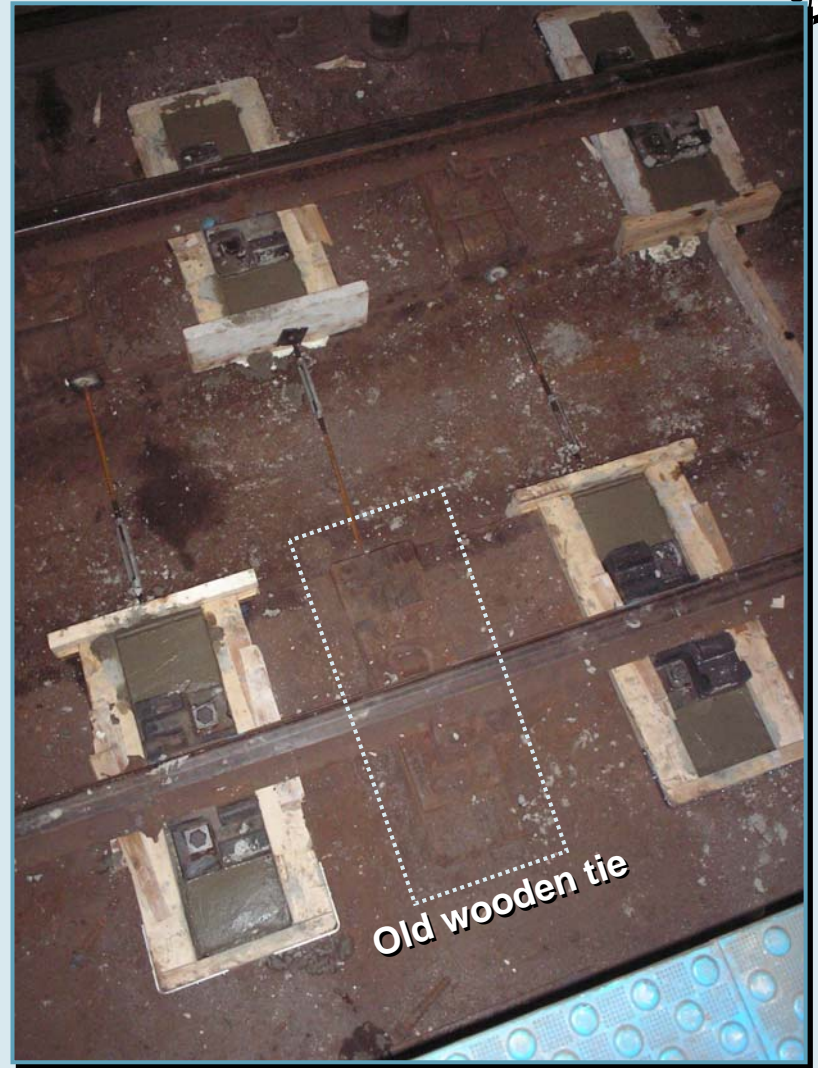
Concrete half-ties curing in their molds
