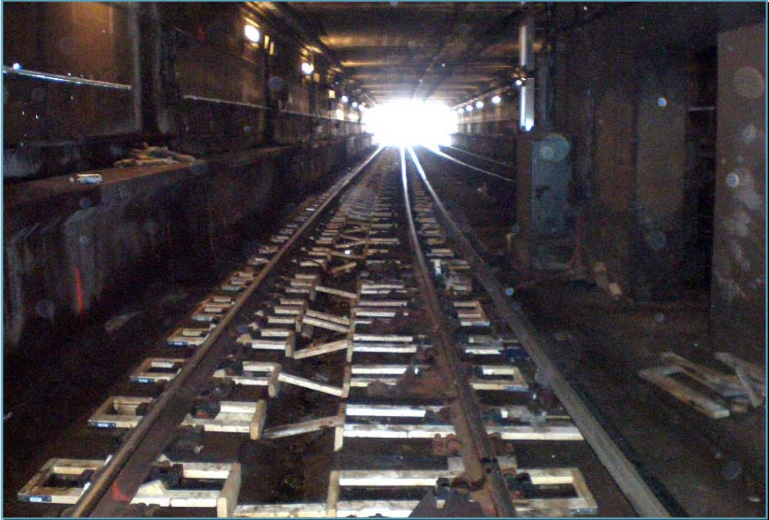
Concrete molds ready for pouring
