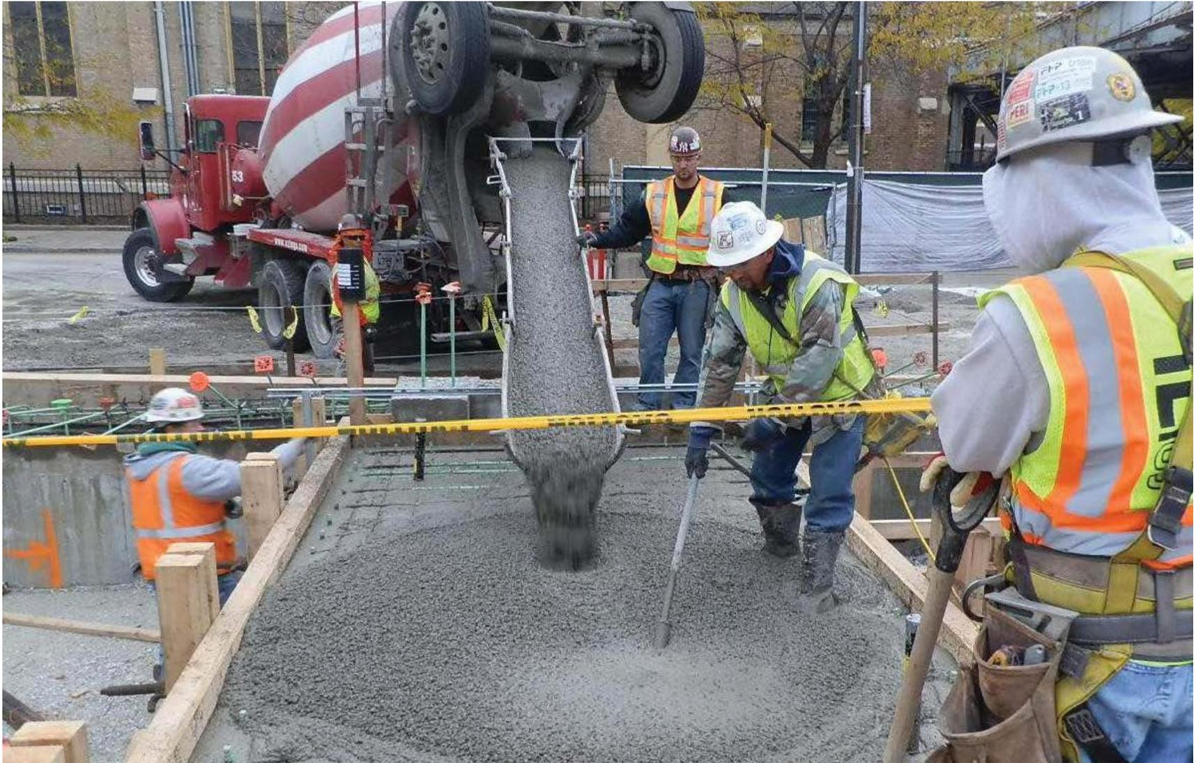
**Hill Substation: transformer pad concrete pour**
