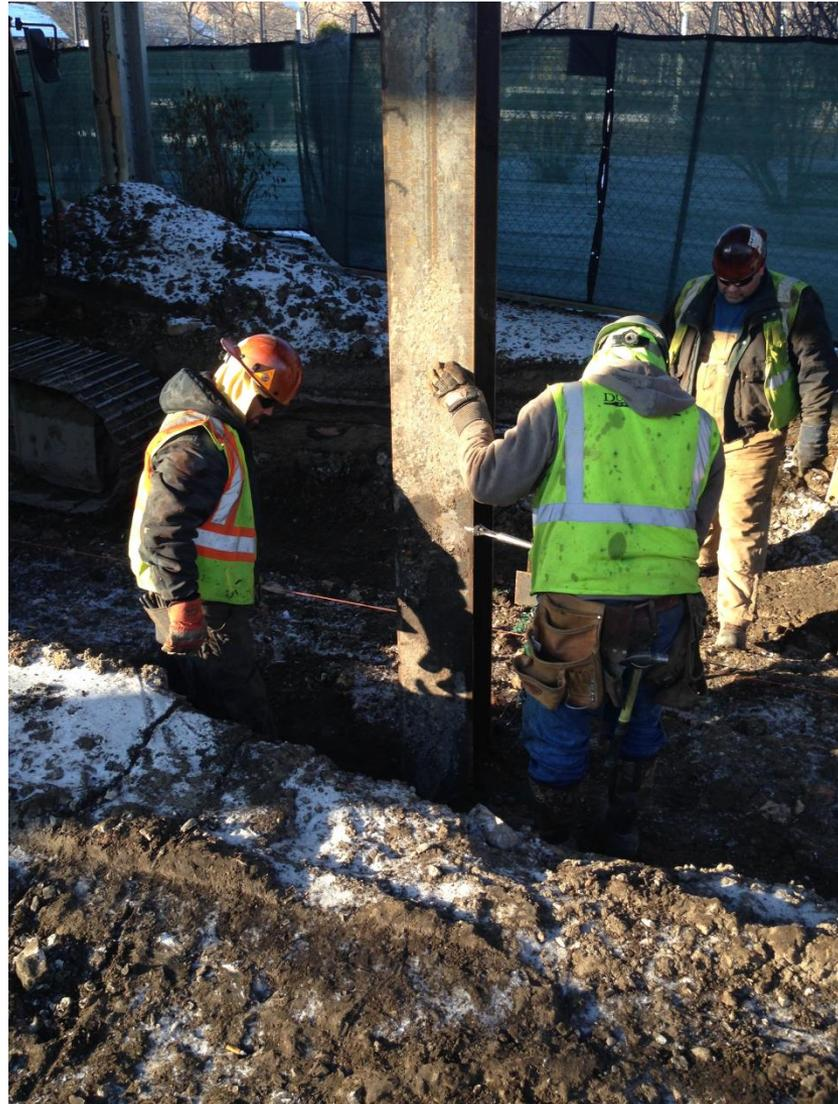
**Hill Substation: H-pile installation for ductbank**
