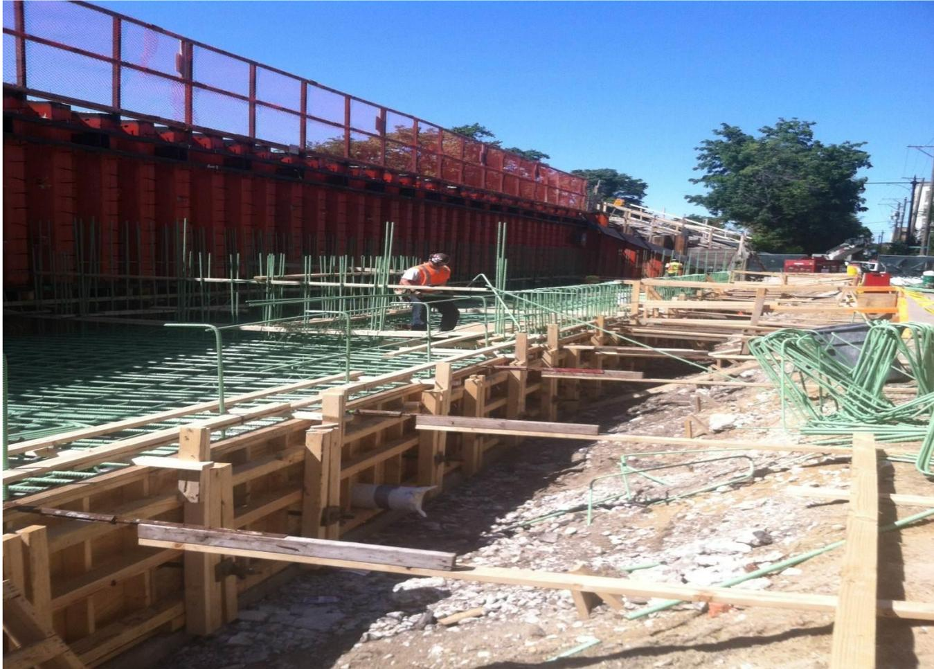
**Contractor installing reinforcing bars for foundation installation at Farwell Substation**
