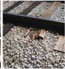
Deteriorated ties and trackbed on the Dan Ryan branch 'L', like these, are requiring slower train speeds and longer trip times.
