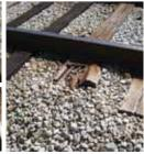
Deteriorated ties and trackbed on the Dan Ryan branch 'L', like these, are requiring slower train speeds and longer
