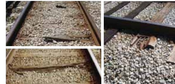
Deteriorated ties and trackbed on the Dan Ryan branch 'L', like these, are requiring slower train speeds and longer trip times.
