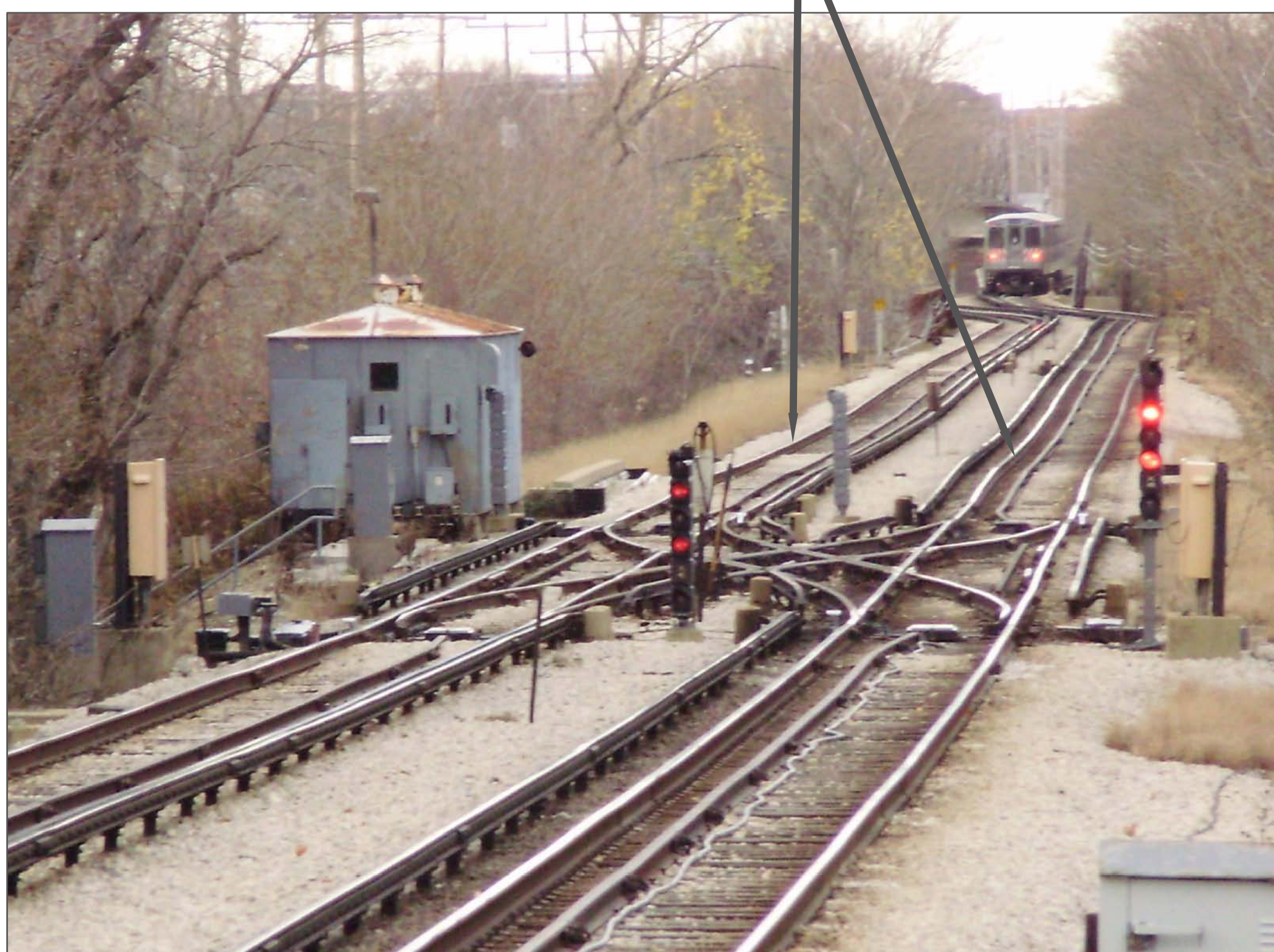
SPECIAL TRACKWORK (DOUBLE CROSSOVER)
