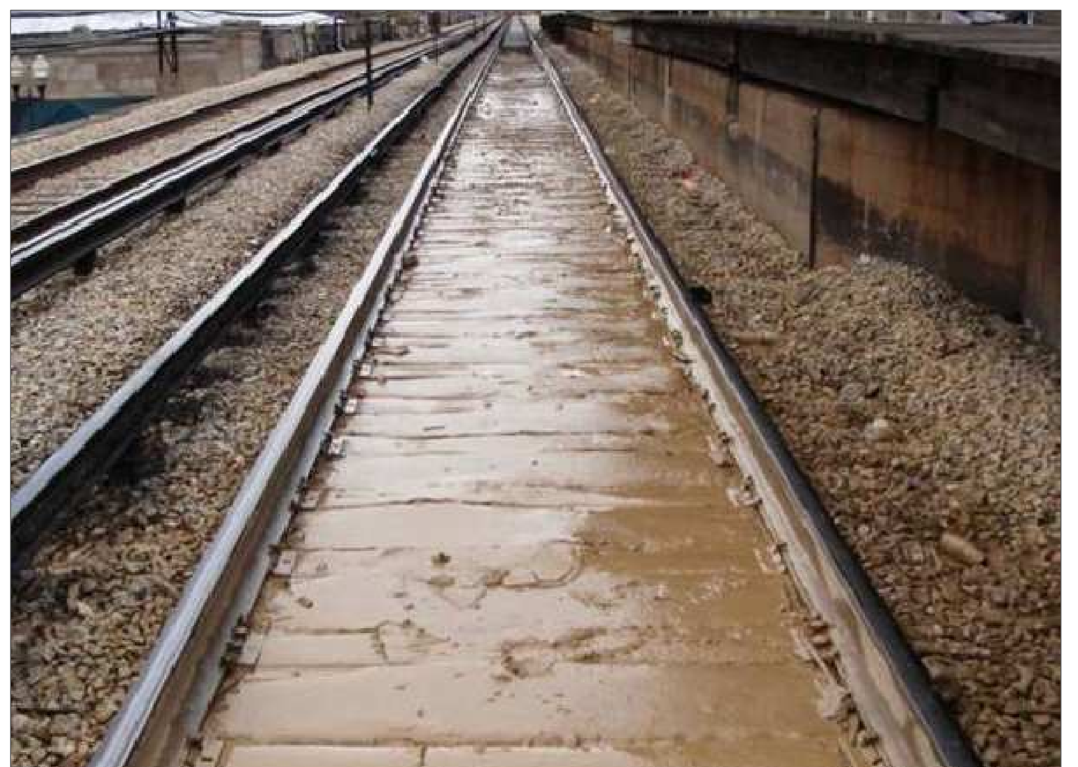
AGING TIES IN WORN BALLAST LACKING DRAINAGE
