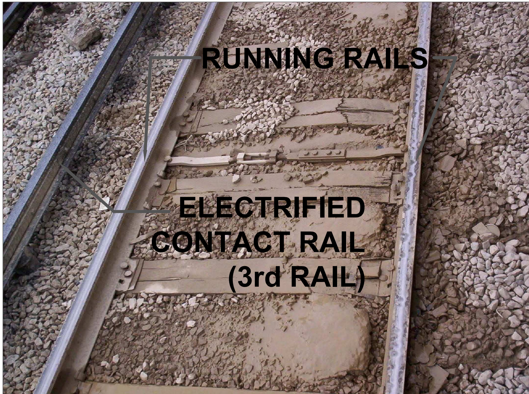
AGING TIES & WORN BALLAST
