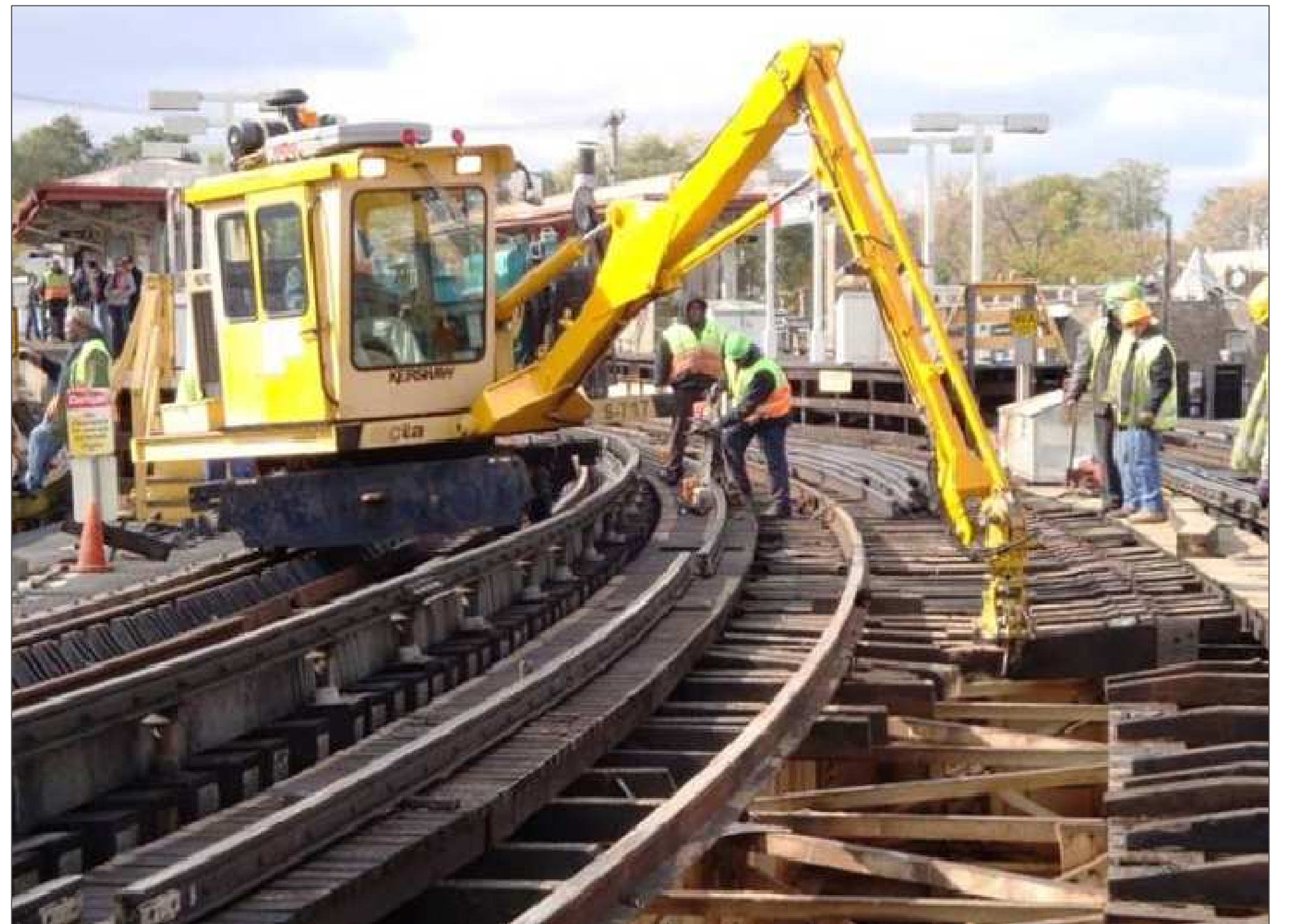
REPLACING AGING OPEN DECK TRACK AND FOOTWALK
