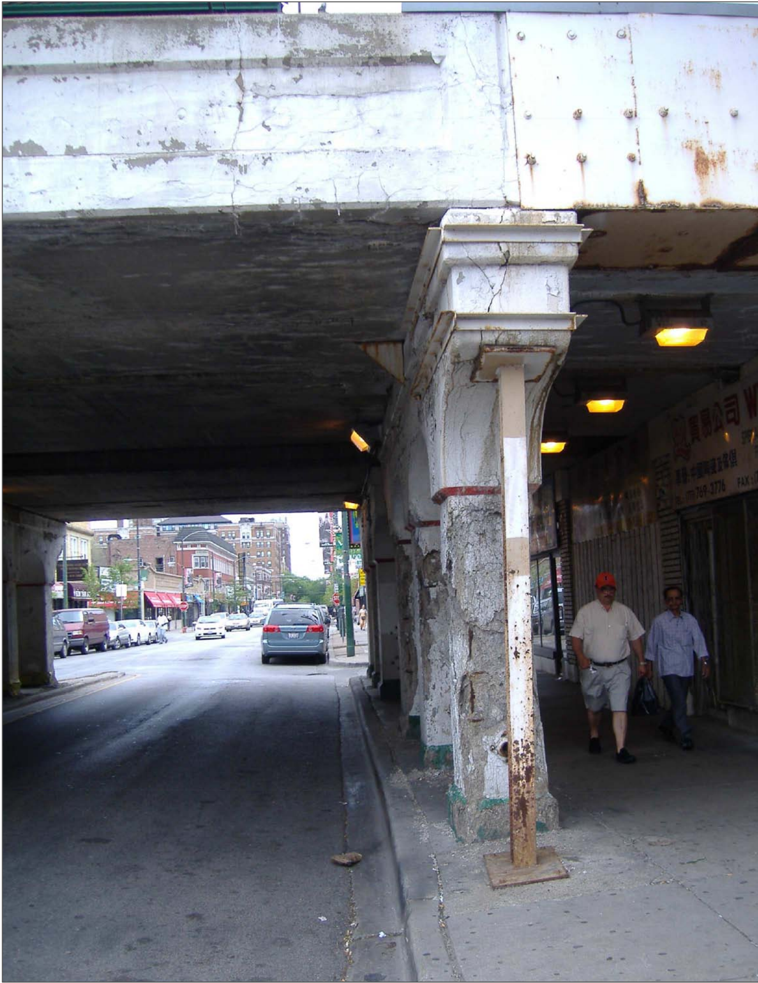
TEMPORARY SUPPORTS OF PIER & PARAPET WALL
