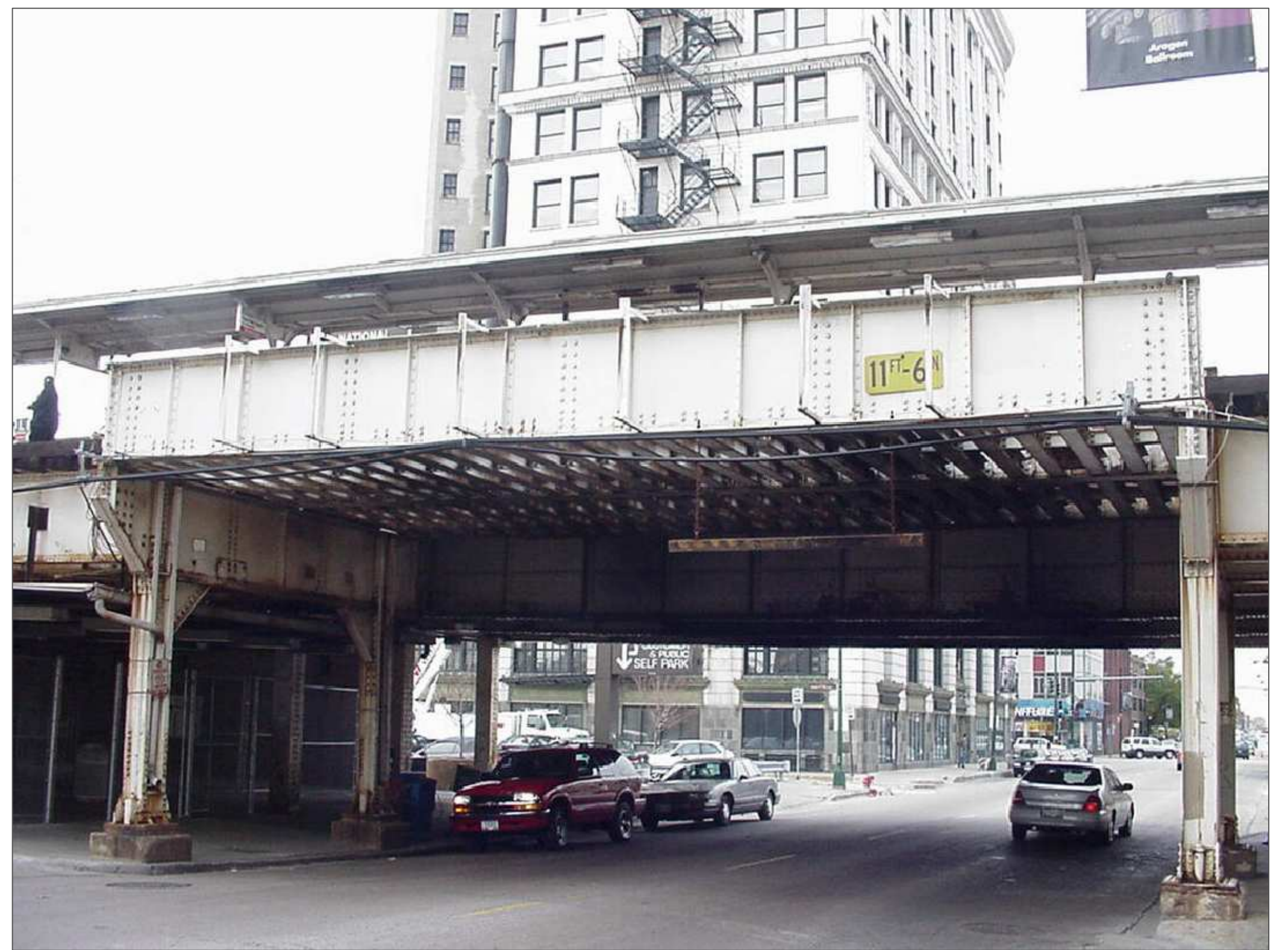
SUBSTANDARD VERTICAL CLEARANCE
