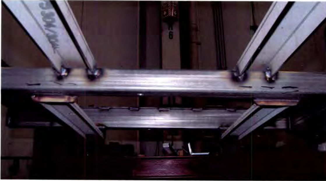
Figure 3: View of underside of wheelchair ramp area showing area to be heated with dashed black lines. This is the tube that is closer to the curb side.
