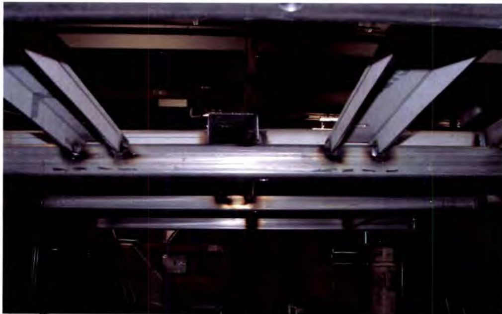
Figure 2: View of underside of wheelchair ramp area showing area to be heated with dashed black lines. This is the tube that is further to the street side.
