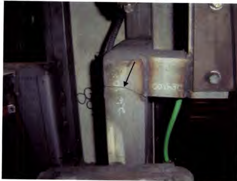
Shown view of cracked A/C L-support bracket that requires to be welded at the defective area.
