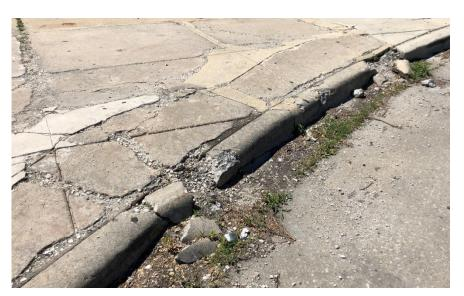
Kedzie (Orange Line) Repairing all broken/cracked curbs at the bus turn-around
