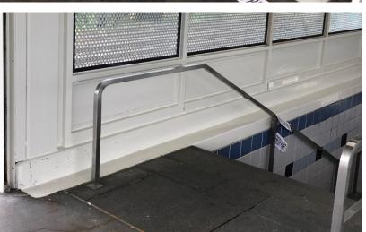
Kedzie (Orange Line) Repaired rusted sections of stairway storefront along with fresh coats of paint and rust inhibitor
