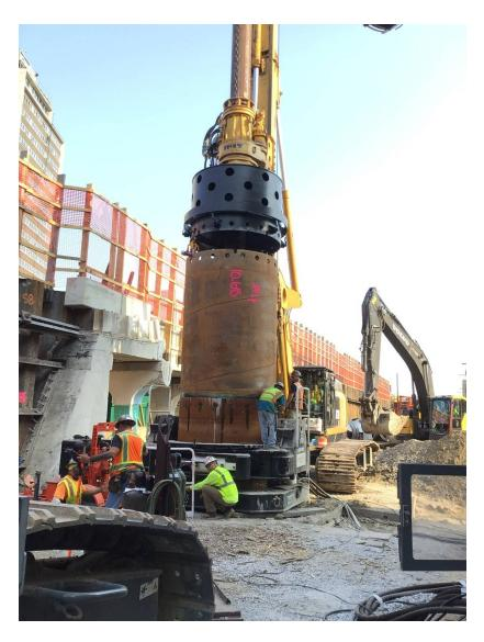
**LBMM – Drilled Shaft Installation**
