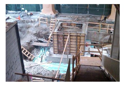
Excavation and forming of elevator foundation
