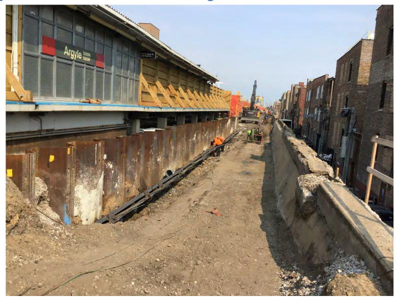
**LBMM – Soil Anchor Installation and Excavation**
