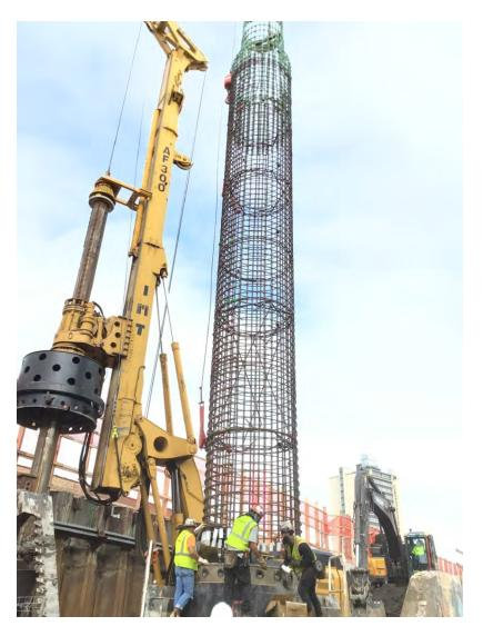
**LBMM – Caisson Rebar Cage Installation**
