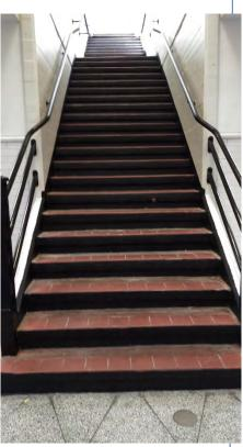
Jarvis (Red Line) Repaired loose stair tiles and painted stair risers and railings
