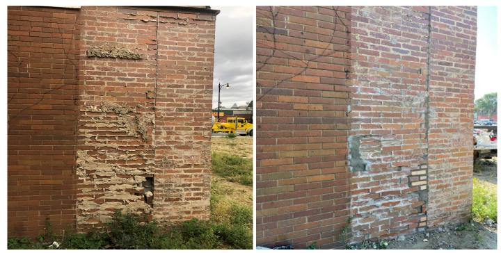
47th (Green Line) Repair & tuckpoint exterior wall of stationhouse
