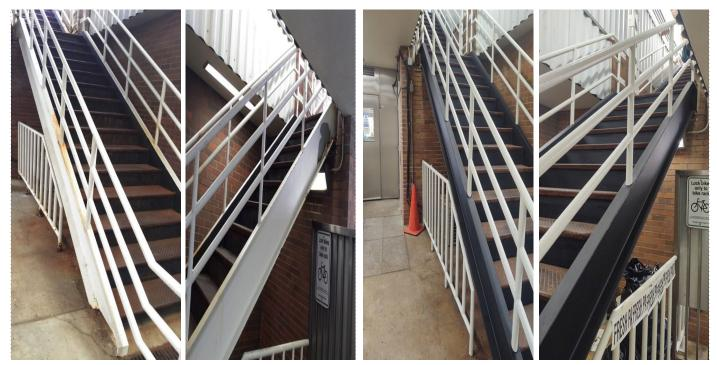
47th (Green Line) Painting of staircase handrails and structure
