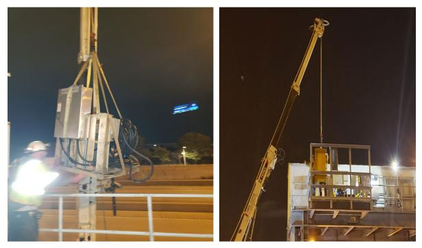
Temp power & Equipment Installation at 87th signal house
