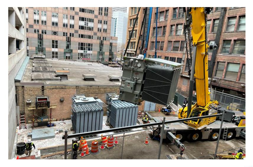
**Hoisting Transformer 1 at Franklin Substation**
