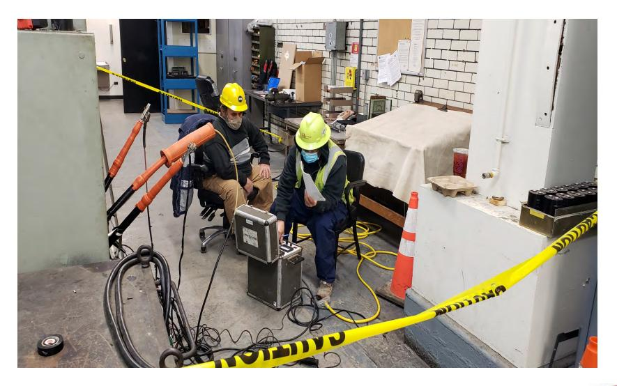
**Feeder Testing of Transformer 1 at Franklin Substation**
