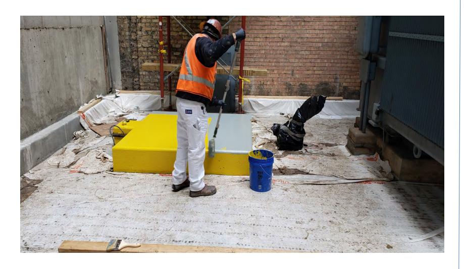
Applying Epoxy Coat over Concrete Pad 1 for Transformer 1 at Franklin Substation
