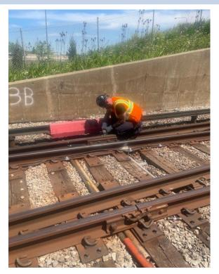
**Prepping Rail for Cadweld Installation at Rosemont West Interlocking**
