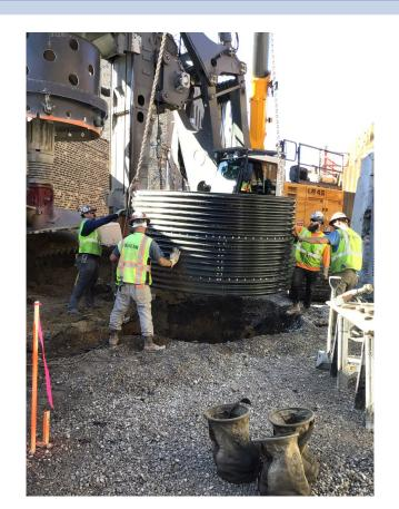
LBMM – Drilled Shaft Installation
