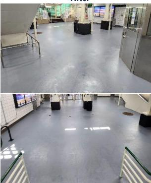
51st/Green Line - Paint station floor with grey epoxy paint
