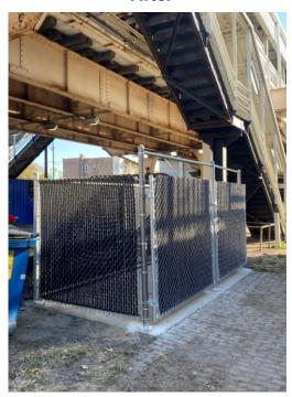
51st Green Line – New location of dumpster Added concrete pad and fencing with privacy slats
