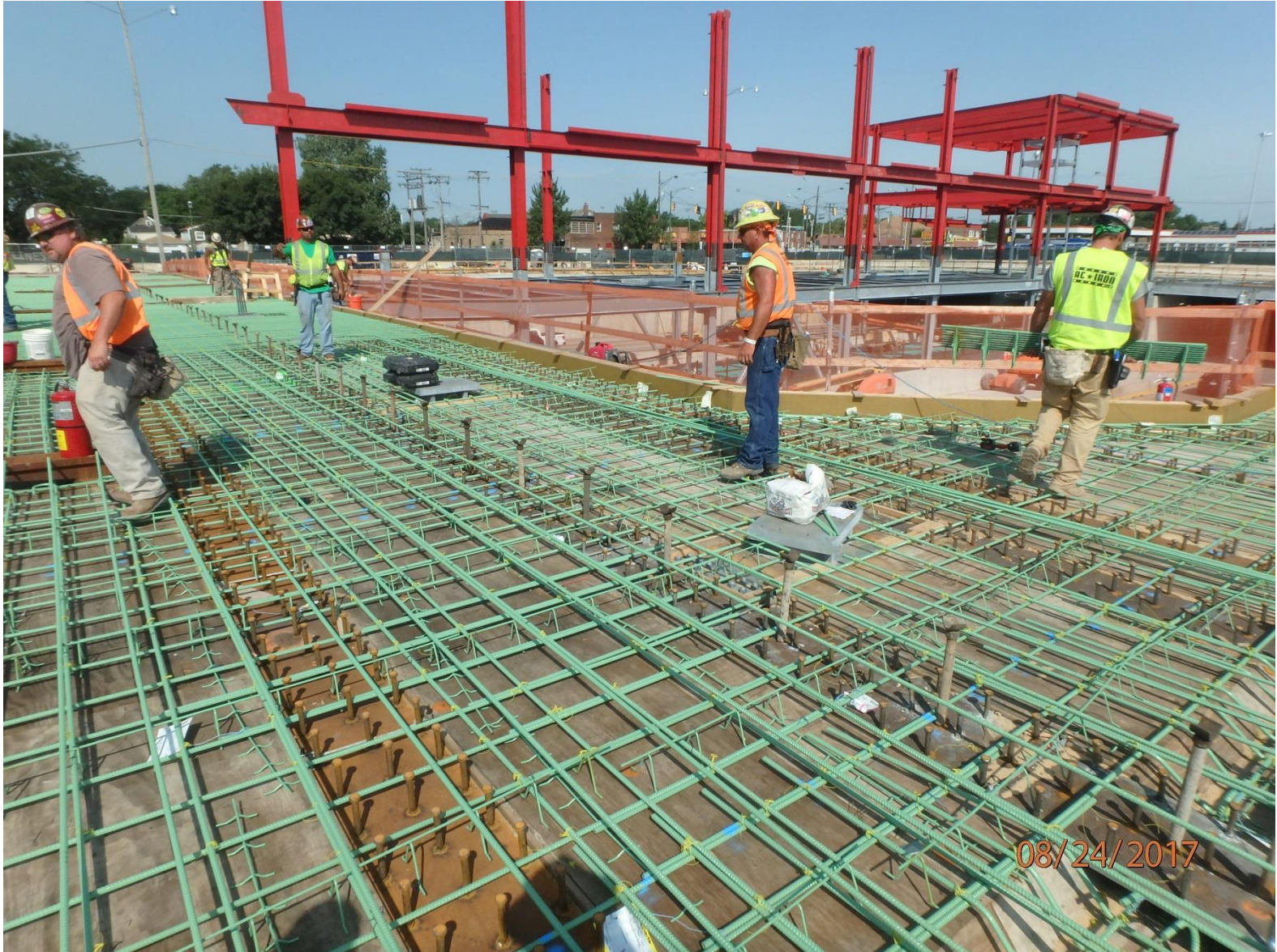
South Bus Bridge Deck - Rebar Installation
