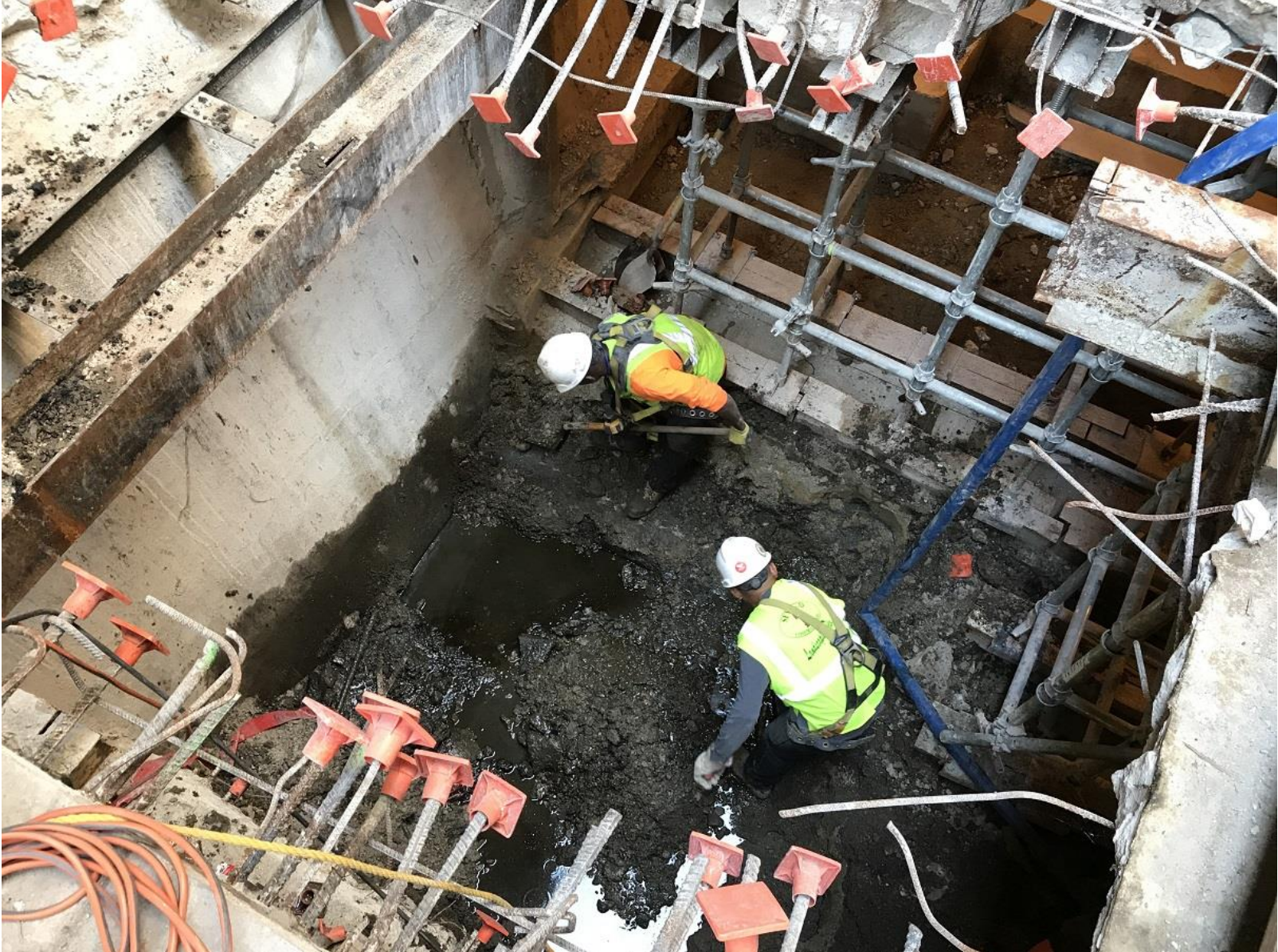
East side – Walkway Column Excavation for New Micropiles
