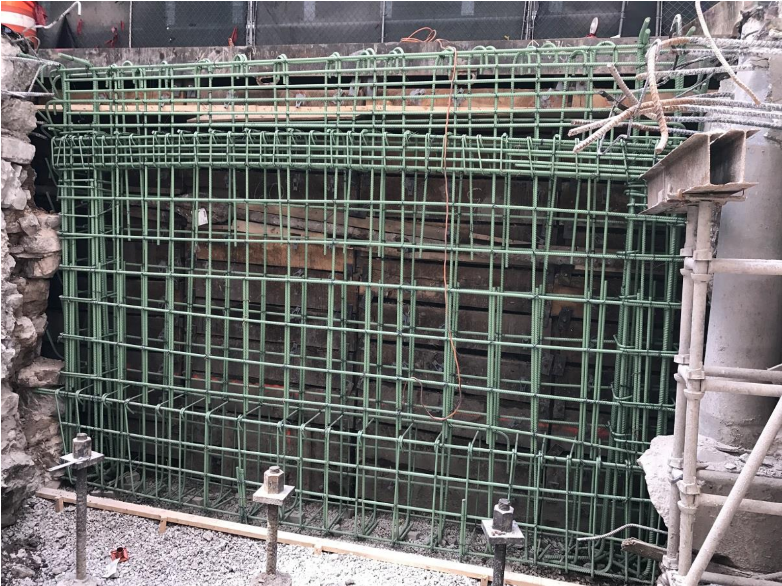
East side – Retaining Wall Rebar Installation at East Elevator Area
