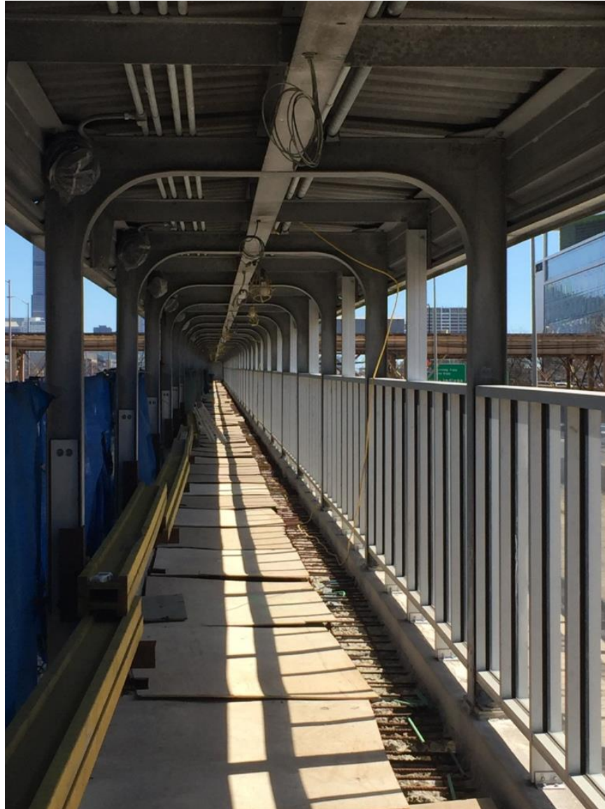
New Storefront Panel installation at Paulina Concourse
