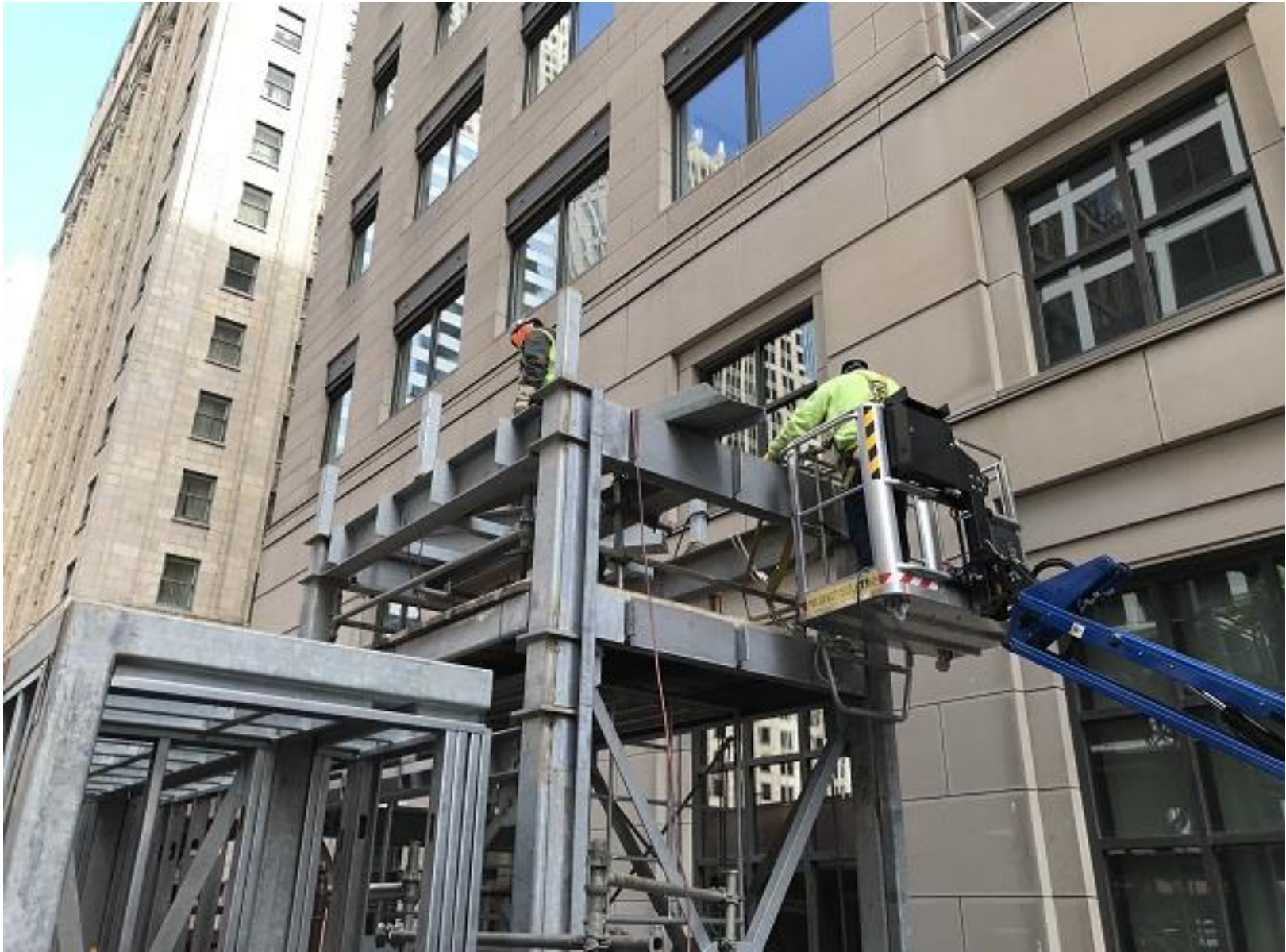
New East Elevator Parapet Steel Installation
