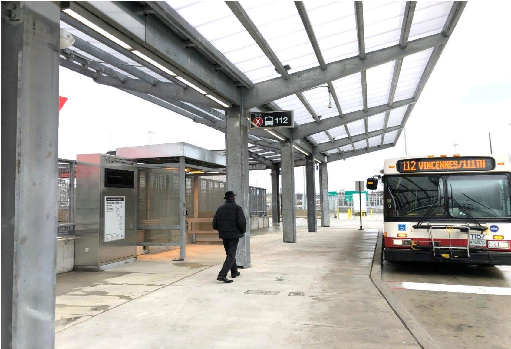
South Terminal: Exterior Bus Area
