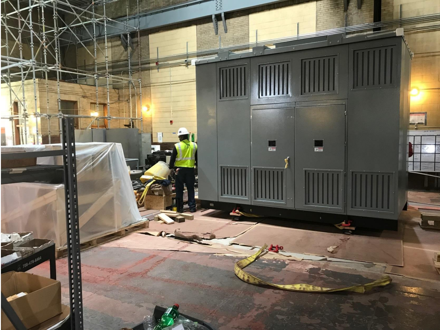
Illinois Substation – Delivery of Transformer
