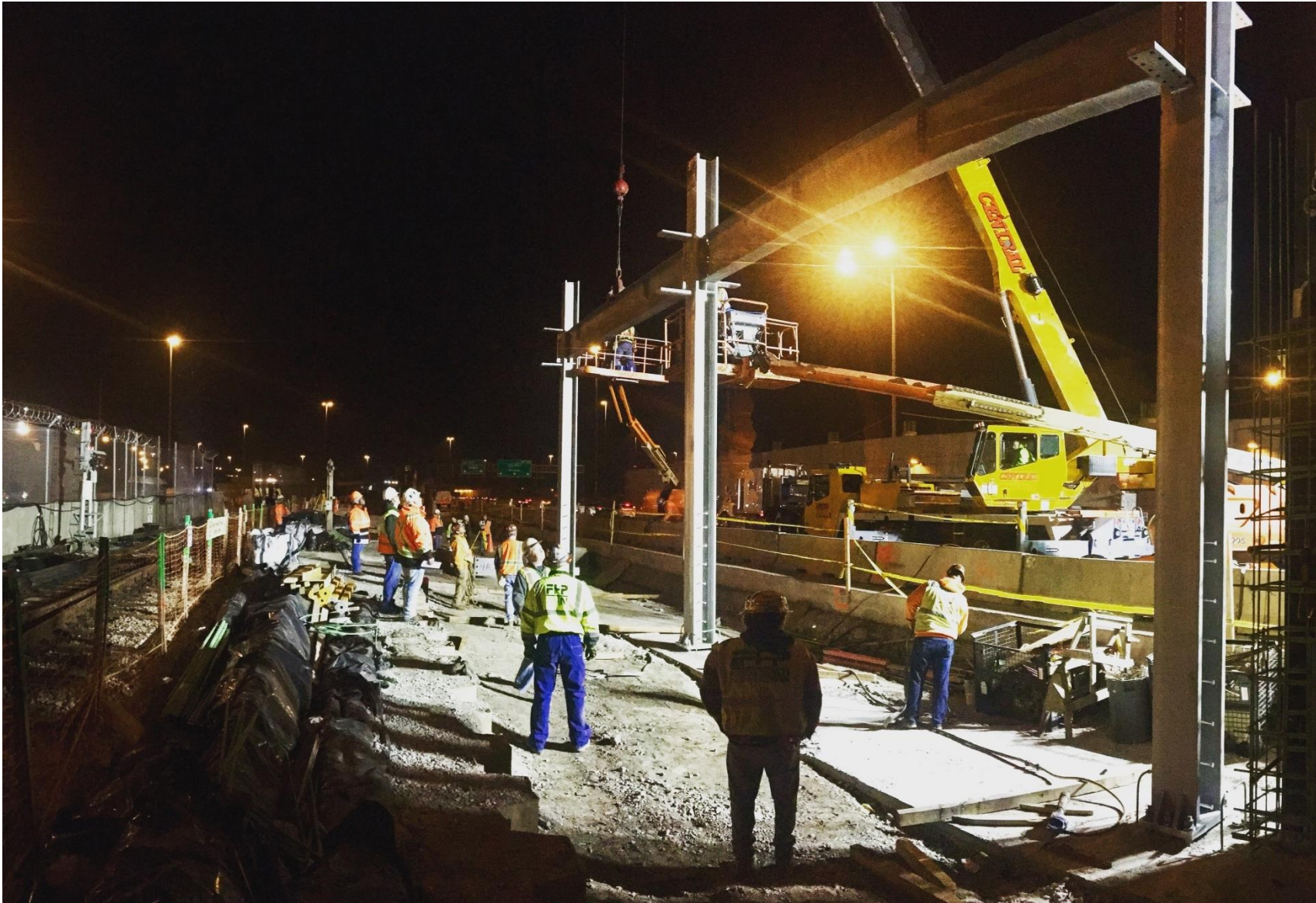
South Terminal Building West Steel Installation
