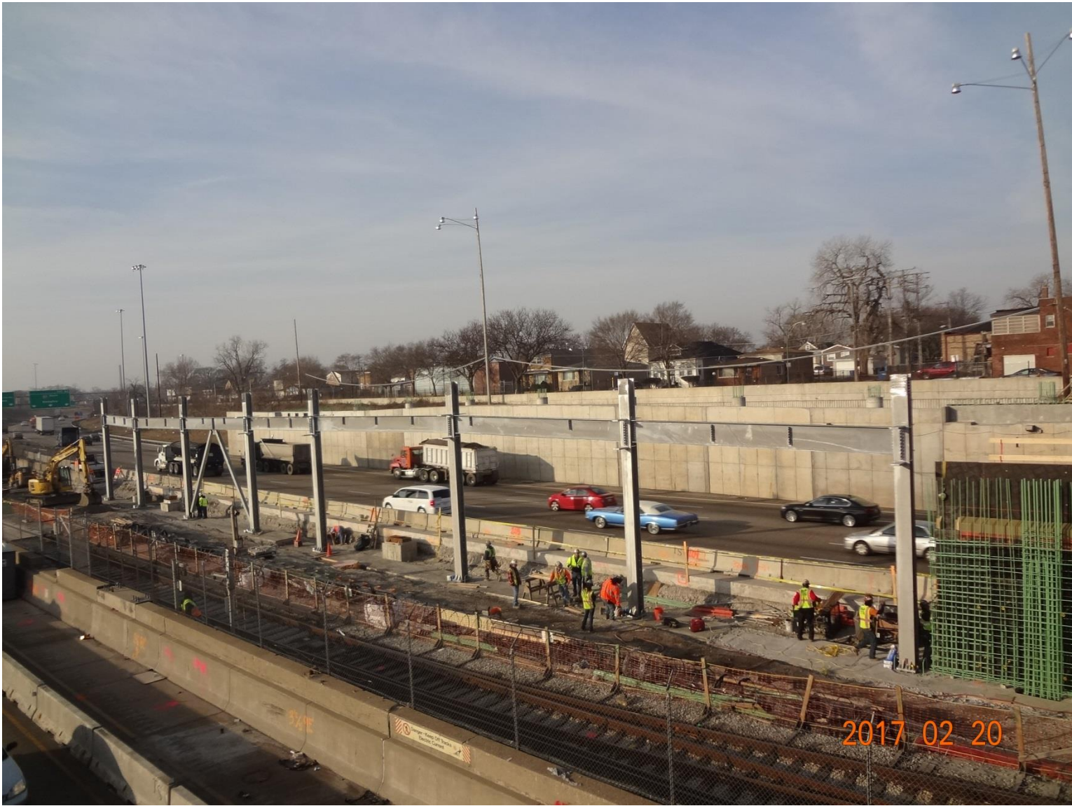
South Terminal Building West Steel Installation
