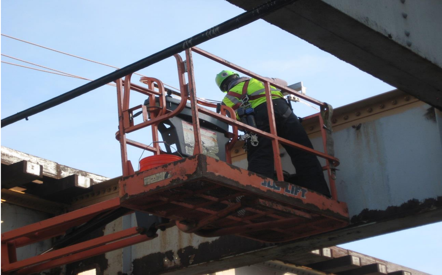
Installation of cable brackets and messenger wire ongoing
