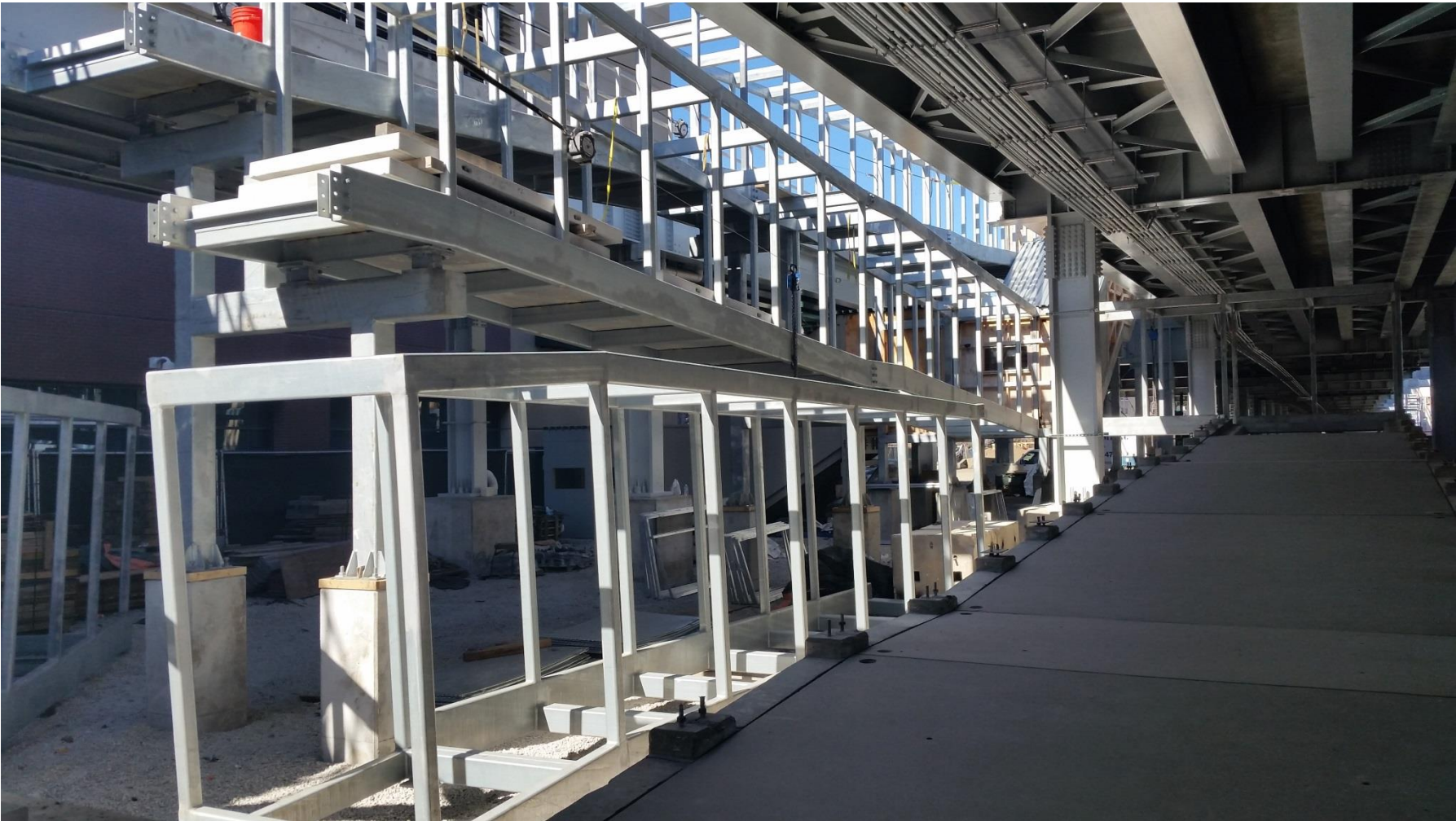
Sunnyside west ramp build out
