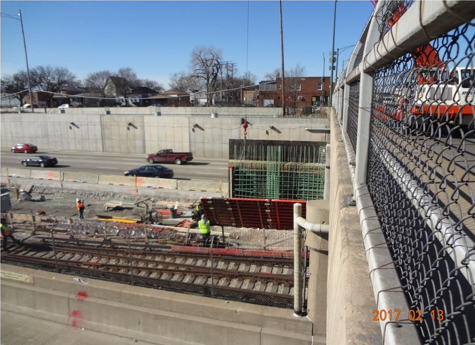
95 th St Bridge Pier Extension Rebar and Formwork Installation
