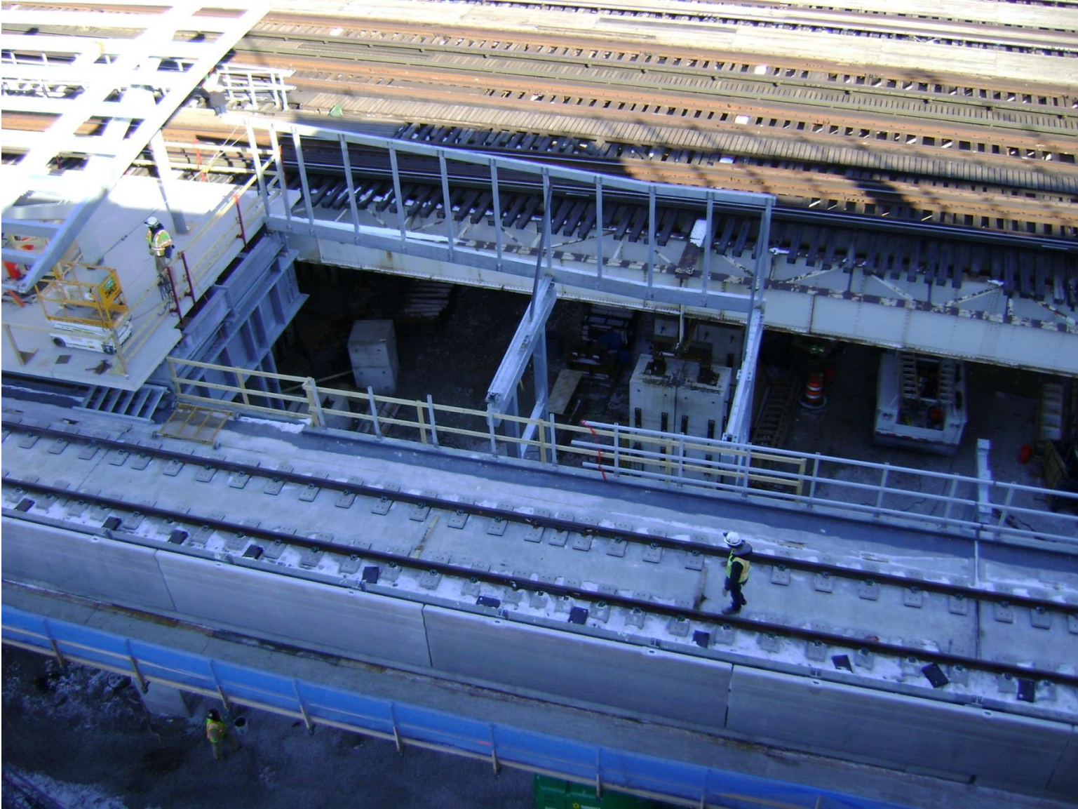
New Sunnyside ramp structure installation
