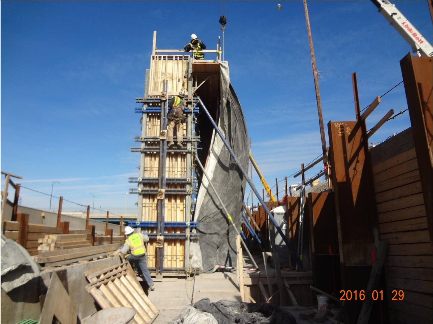
Concrete wall work in southeast corner
