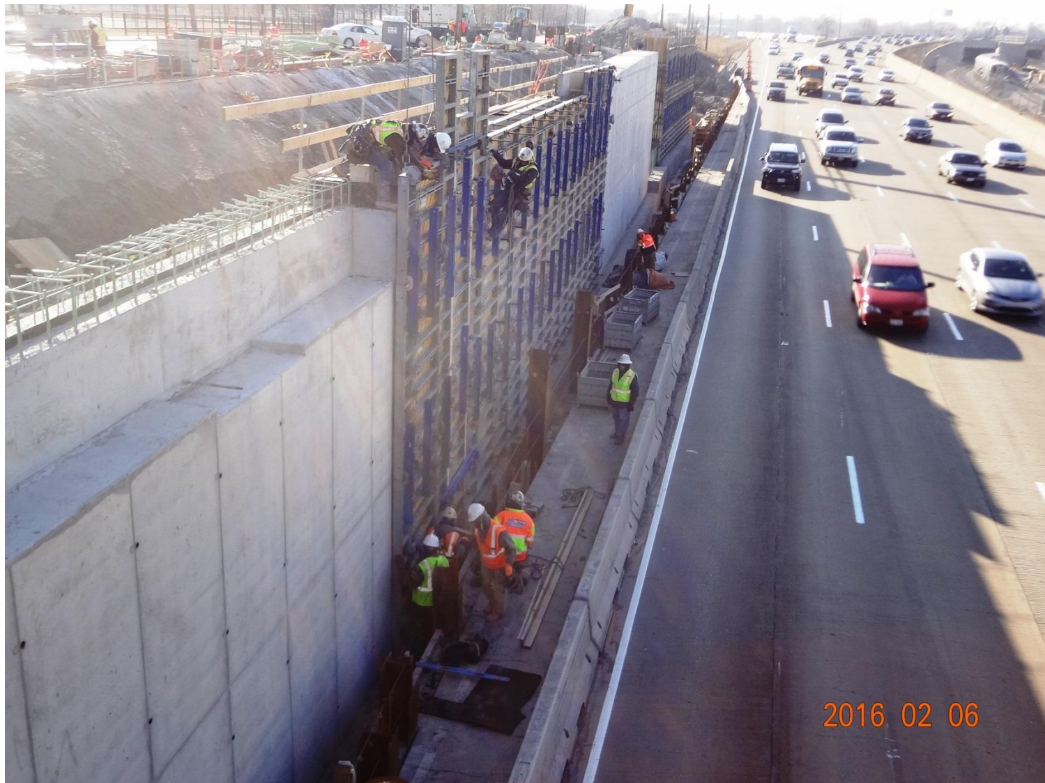
Concrete wall work in southeast corner
