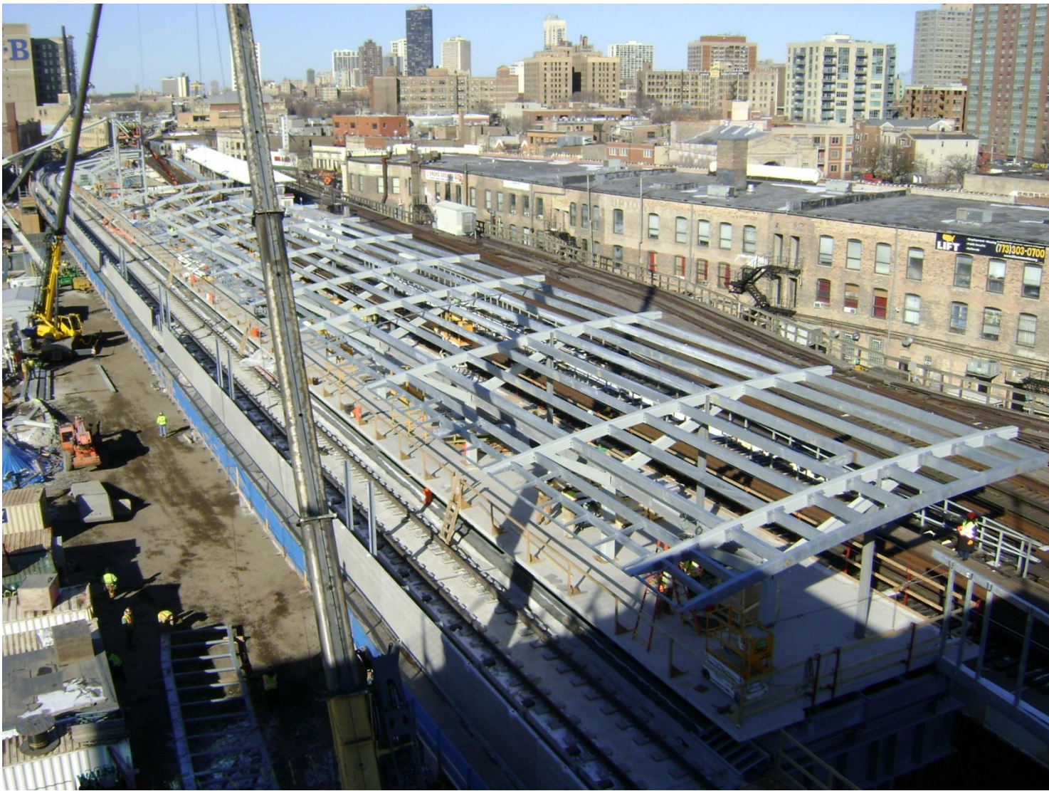
New platform canopy installation
