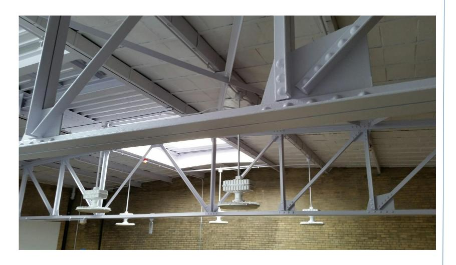
Illinois Substation – Painted Ceiling and Steel with new light fixtures and fire alarm system
