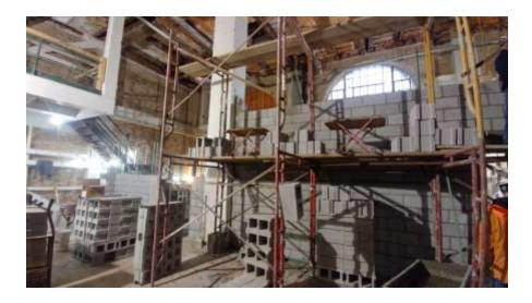
Interior CMU Wall Installation at East Lake Substation
