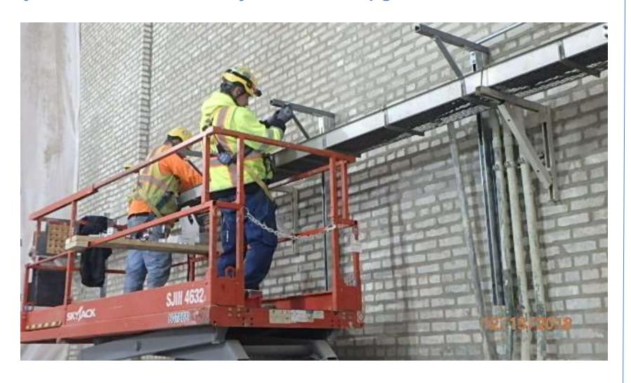
Installation of Bracket Supports for Cable Trays and Conduit
