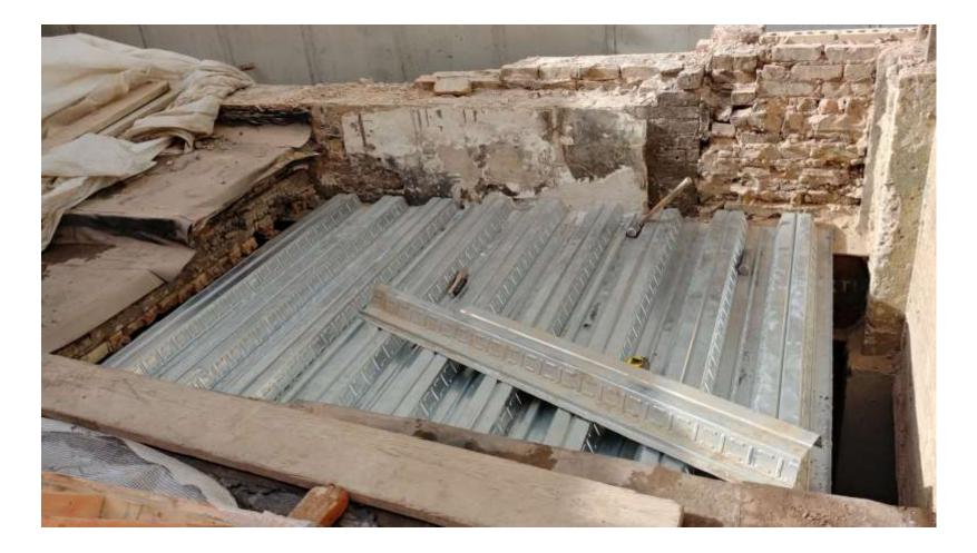
Metal Decking Installation at East Lake Substation
