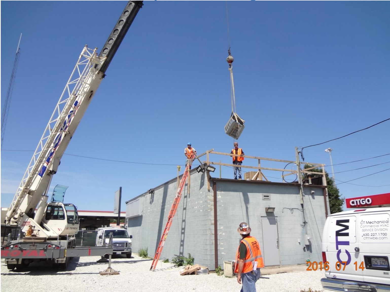
Contractor Field Office Set-Up Work
