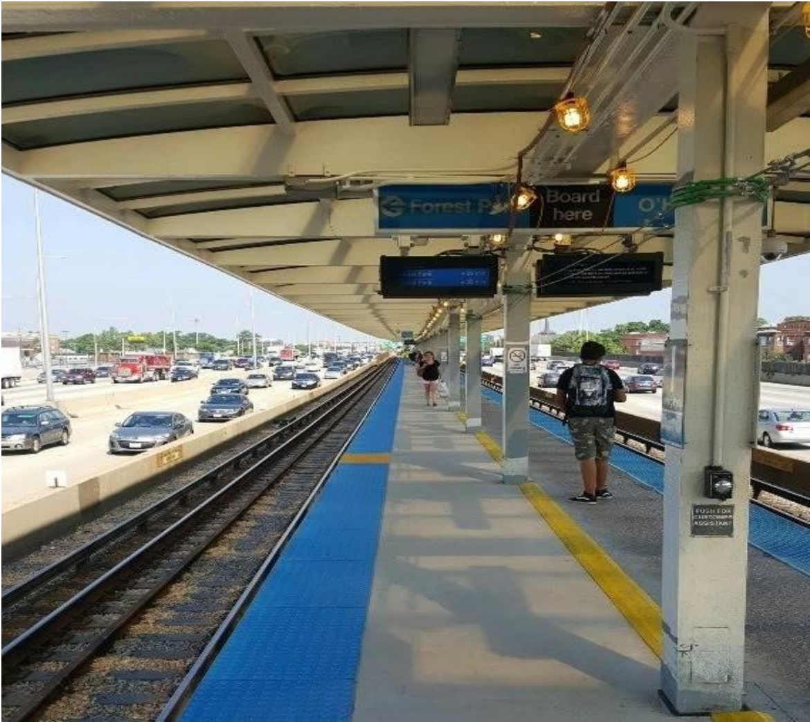
New southbound platform at Irving Park
