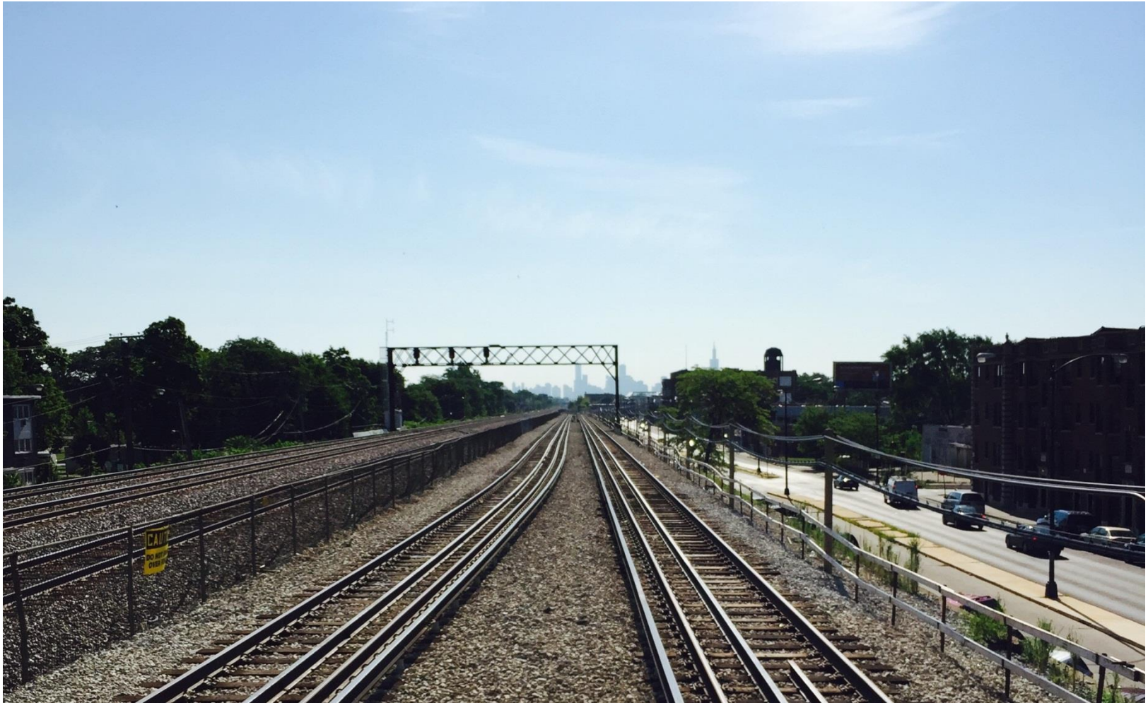
Completed Trackwork – Near Central Station (Facing East)
