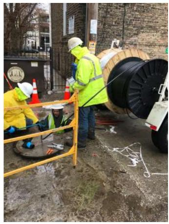
Base to Grade Finish Installation around AT&T manhole on Clark Street (left) and RCN innerduct installation in RPB area (right)
