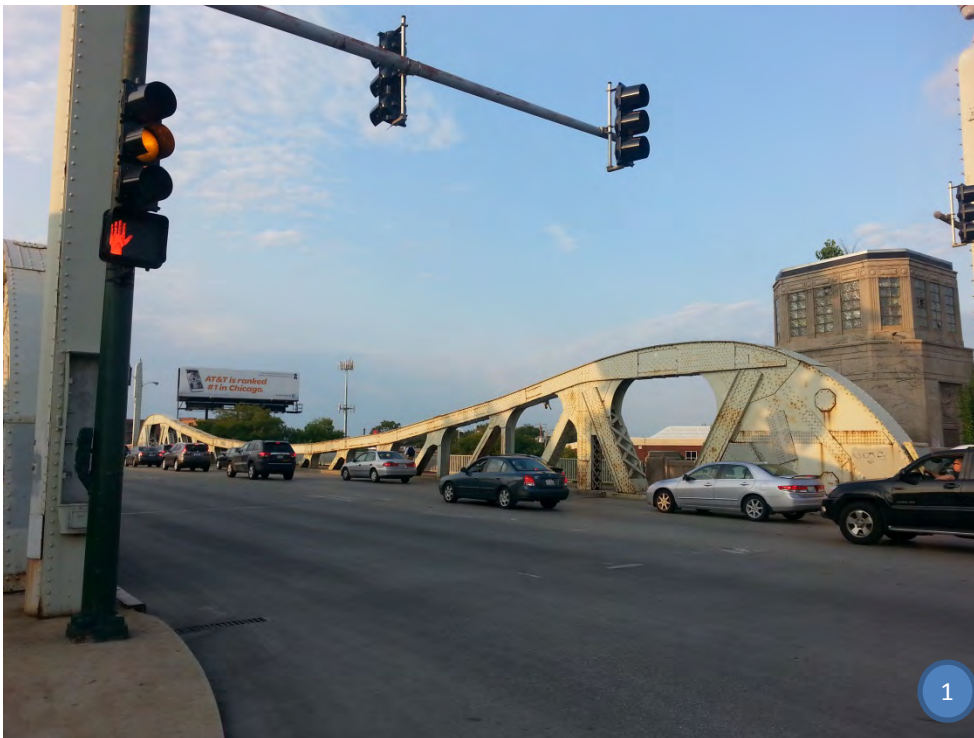
North Ashland Avenue Bridge
