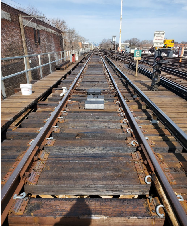
SB Track South of 61 st Interlocking Tie Renewal
