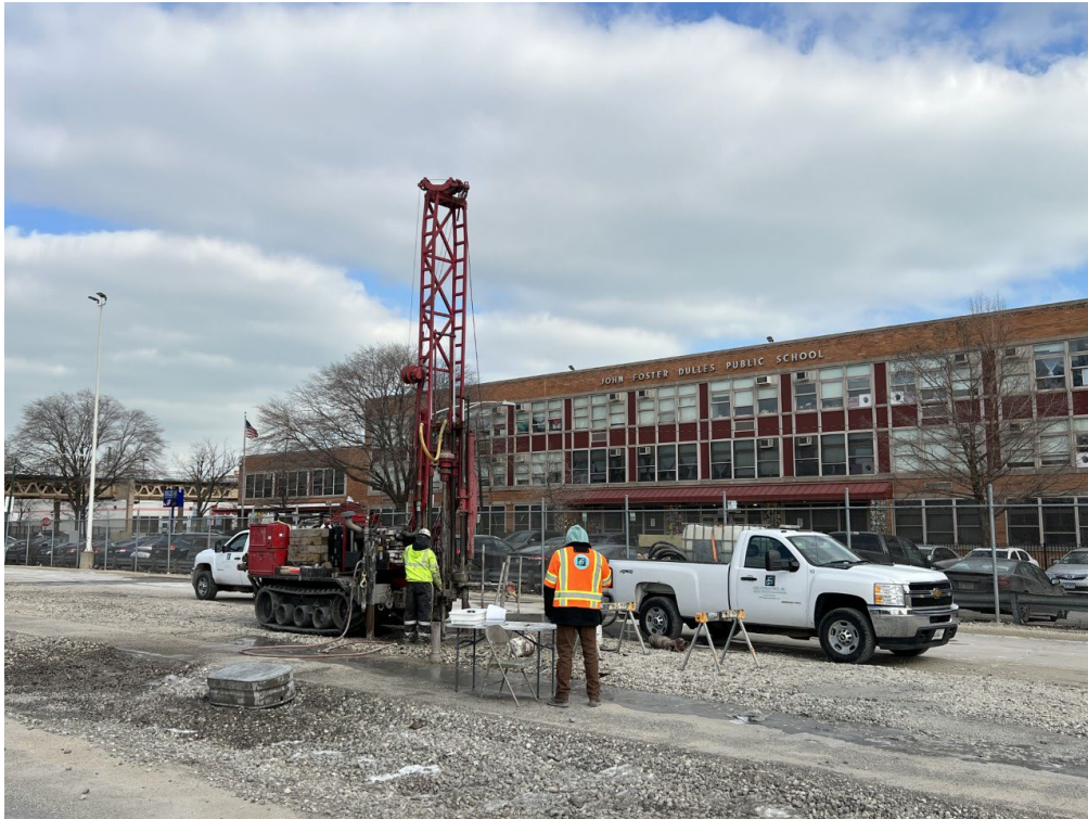
Rock Coring Process
