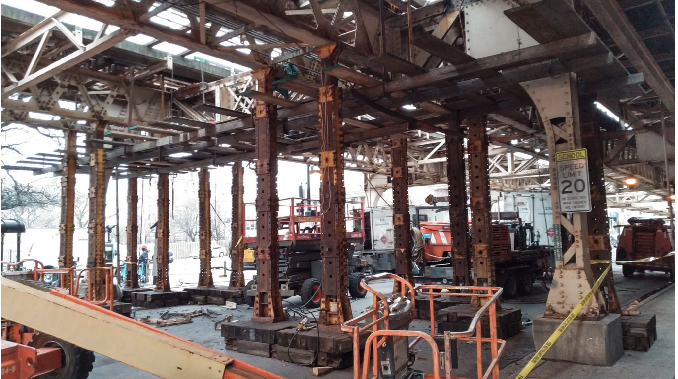
Cross Girder Replacement
