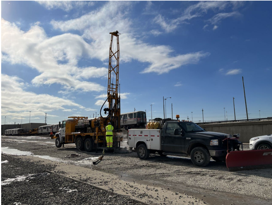
Rock Coring Rig
