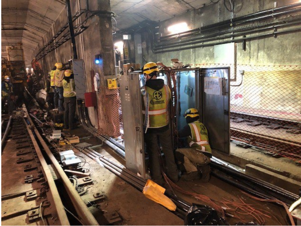
Wiring of Junction Boxes at O'Hare East
