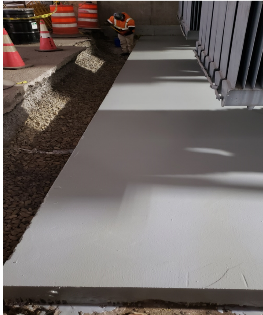
Finished Layer of Epoxy
