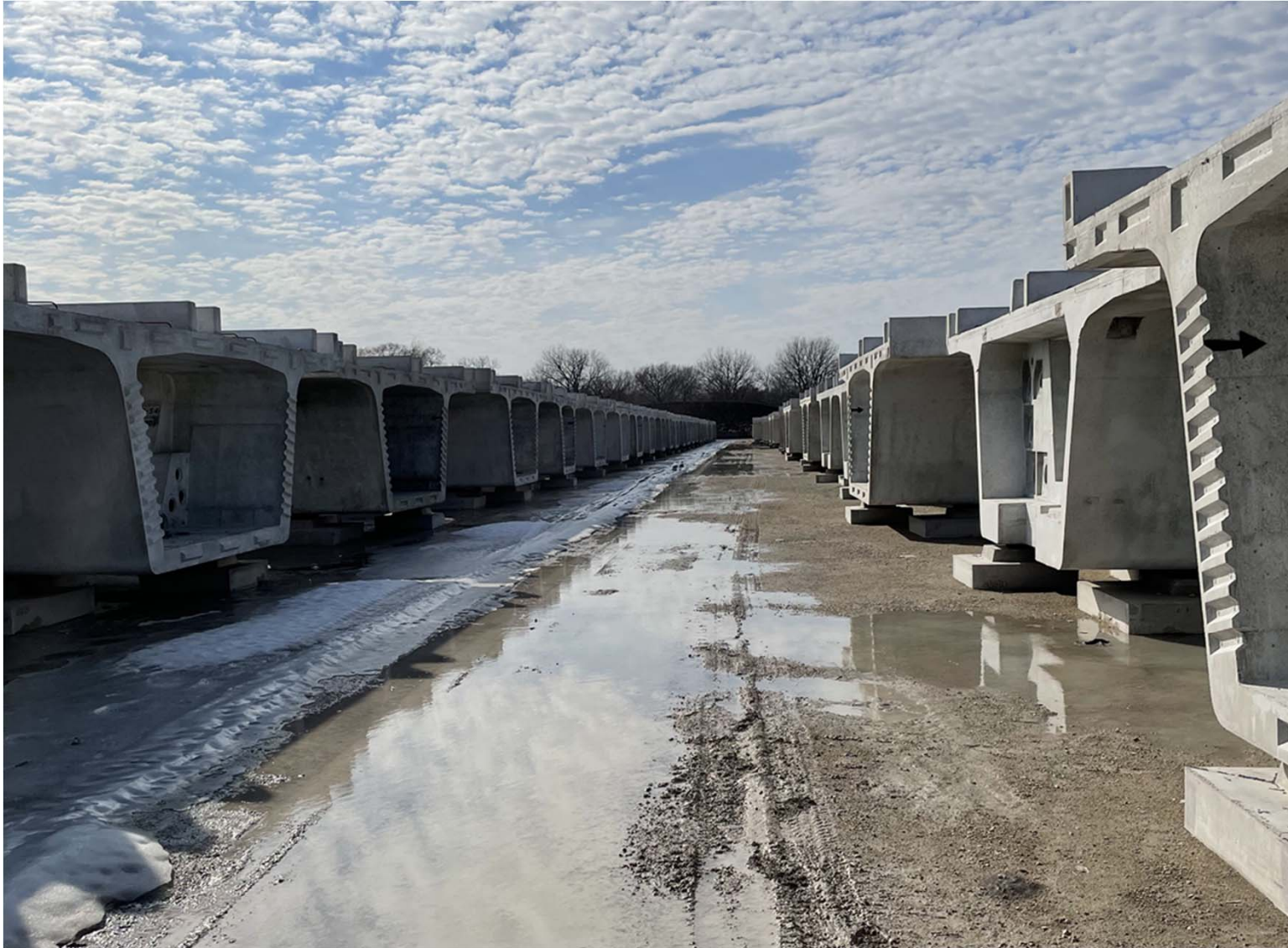
LBMM – Box Girder Segments in Storage
