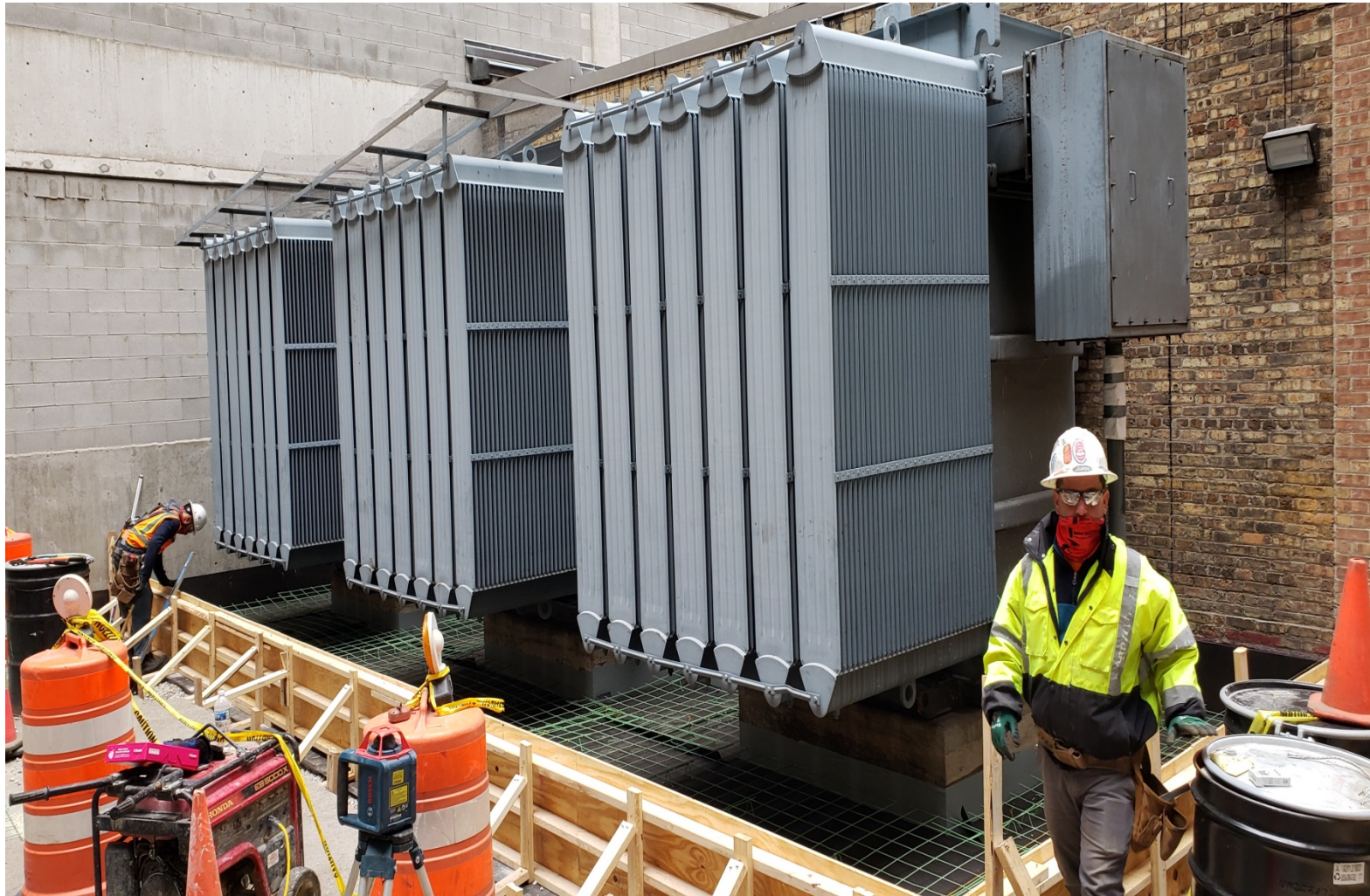
Forming and Reinforcement of the Containment Pad
