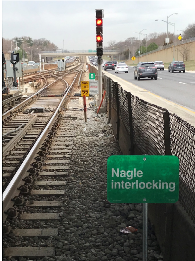
Nagle Interlocking and Signage
