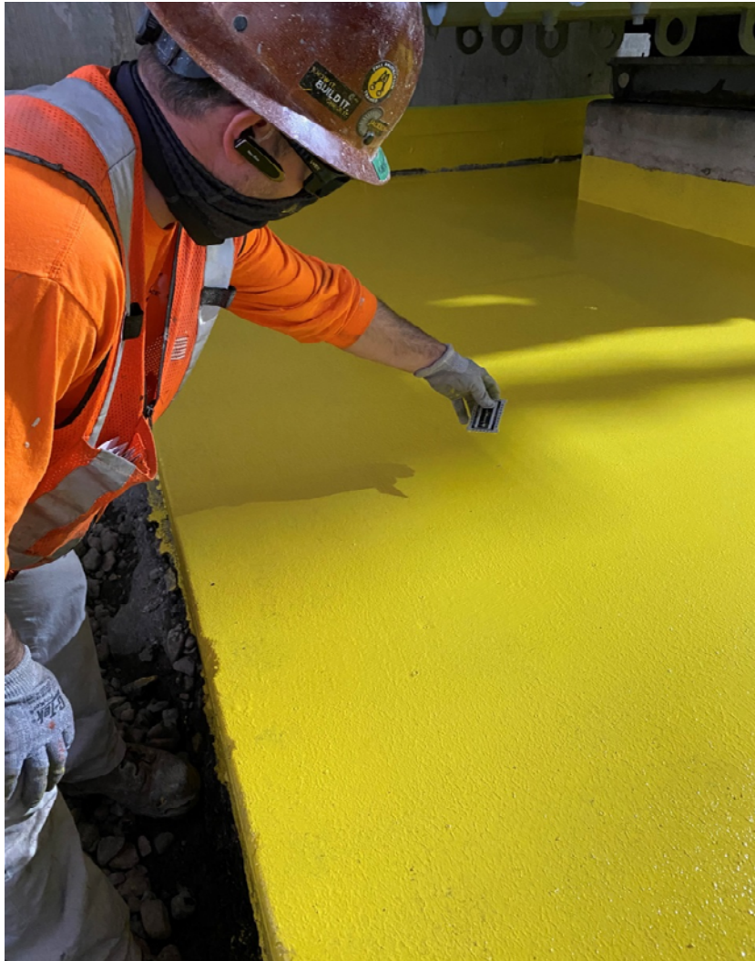
Epoxy Coat 1 - Mil Test
