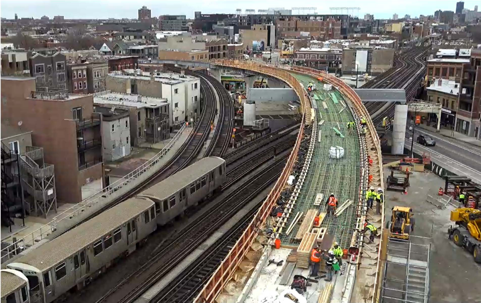
RPB – Constructing Flyover Deck
