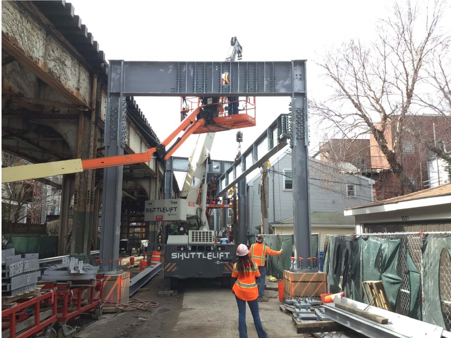
RPB – Flyover Track Structure in Newport / Roscoe Alley
