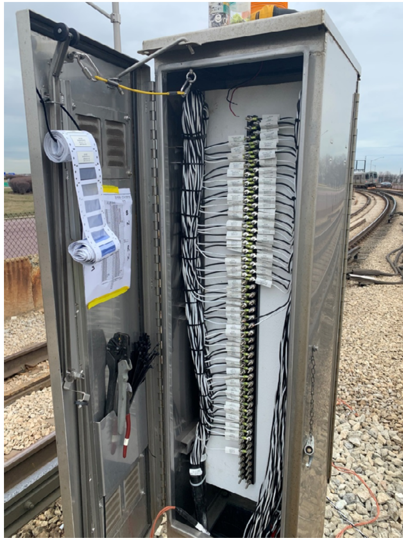
Old Mannheim Junction Box Installation and Wiring
