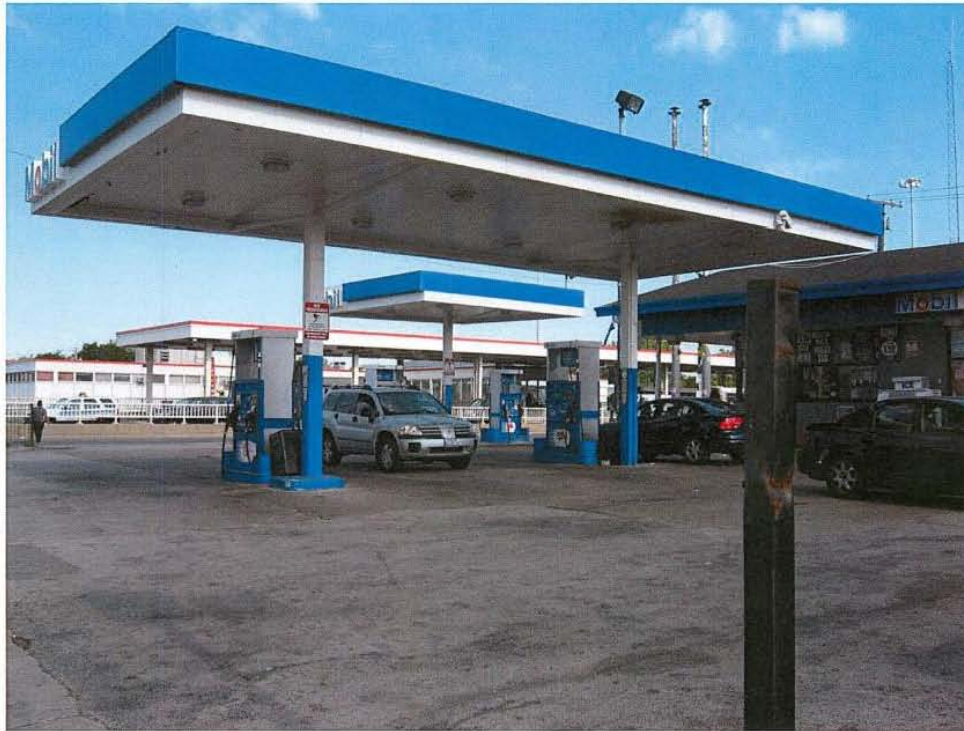
LOOKING NORTHEAST AT THE SUBJECT PROPERTY
