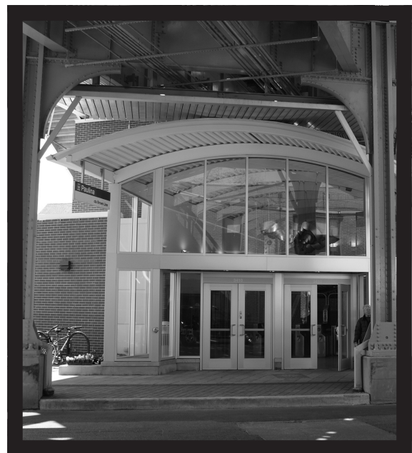
The Paulina Brown Line station was the 15th of 18 stations to be renovated as part of the Brown Line capacity expansion project.
