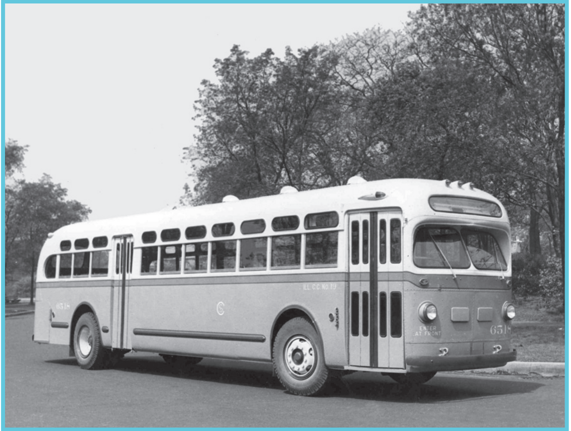
Chicago Surface Lines (CSL) bus #6518, manufactured by General Motors Corporation (GMC) in 1946, has just arrived from the factory at the time of this photo. By today's standards, these buses were extremely basic, and were equipped with manual transmissions, making their operation quite a challenge from an operator standpoint.
