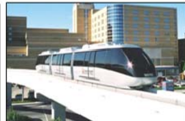
Clarian Automated Guideway Transit
