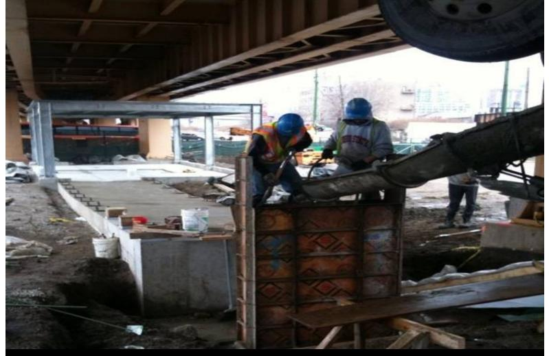
Concrete walkway poured and footing for staircase being prepped for installation.
