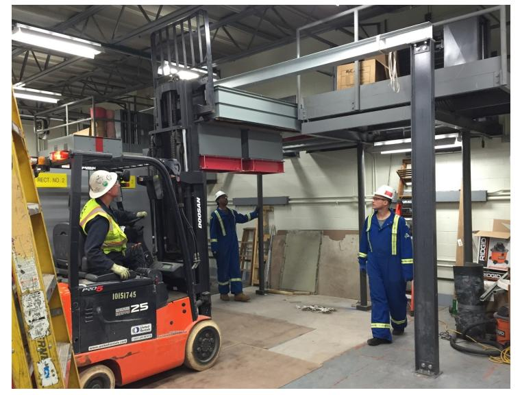
**Princeton Substation: Installation of New Bus Duct**
