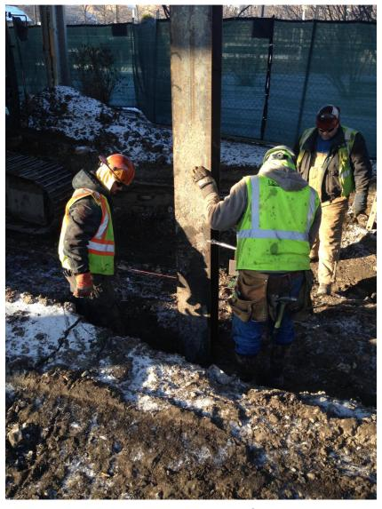
Hill Substation: H-pile installation for ductbank
