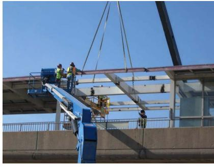
Platform concrete removal to accommodate new escalator, stair and new walkway to south Cermak.
