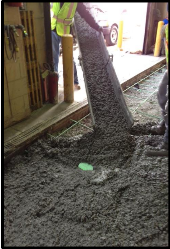
South Shops Garage – Pouring Concrete Floor Slab and Installing Lift Equipment
