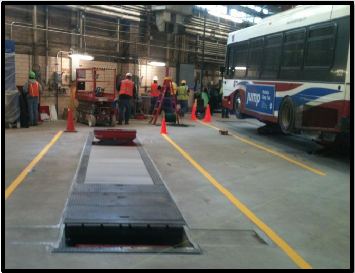
Forest Glen Bus Garage – Installing Floor Slab and Installing /Testing Lift Equipment
