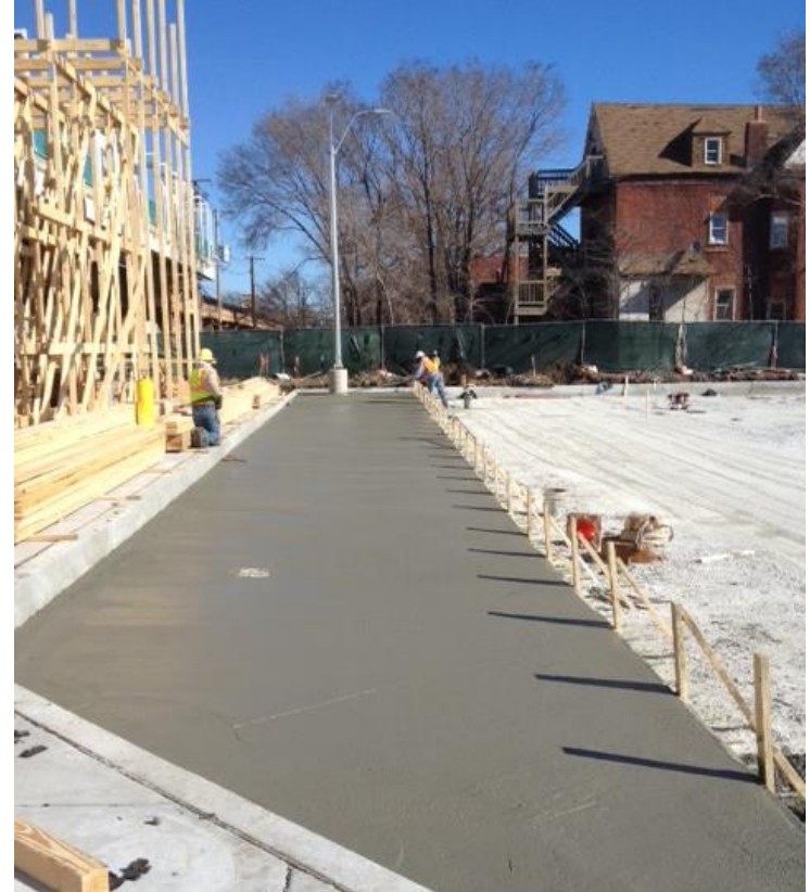
Garfield Station: Bus Lot Being Poured and Auxiliary Stairs Being Built
