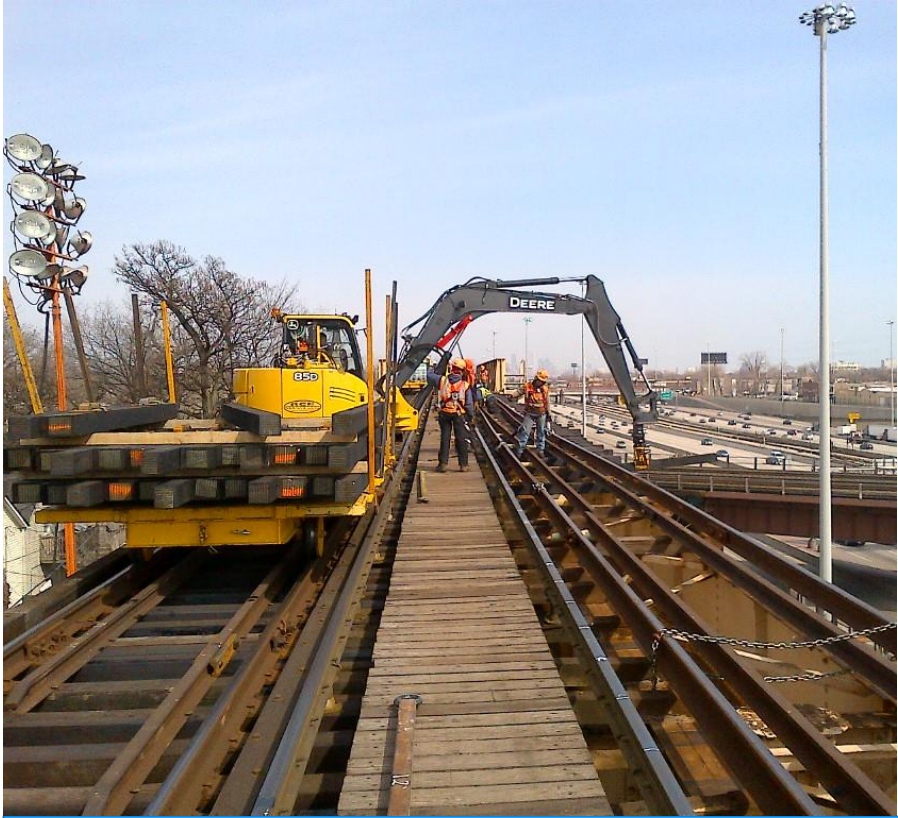
Englewood Track Renewal
