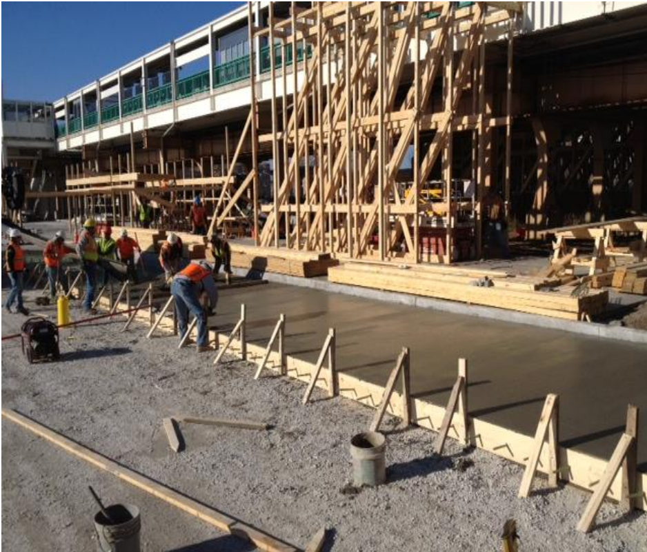
Garfield Station: Bus Lot Being Poured and Auxiliary Stairs Being Built
