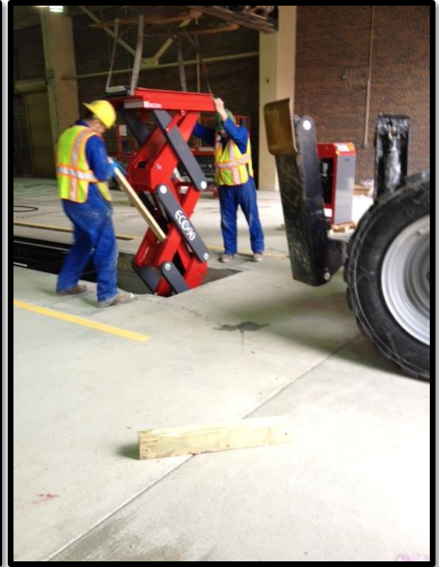
South Shops Garage – Pouring Concrete Floor Slab and Installing Lift Equipment
