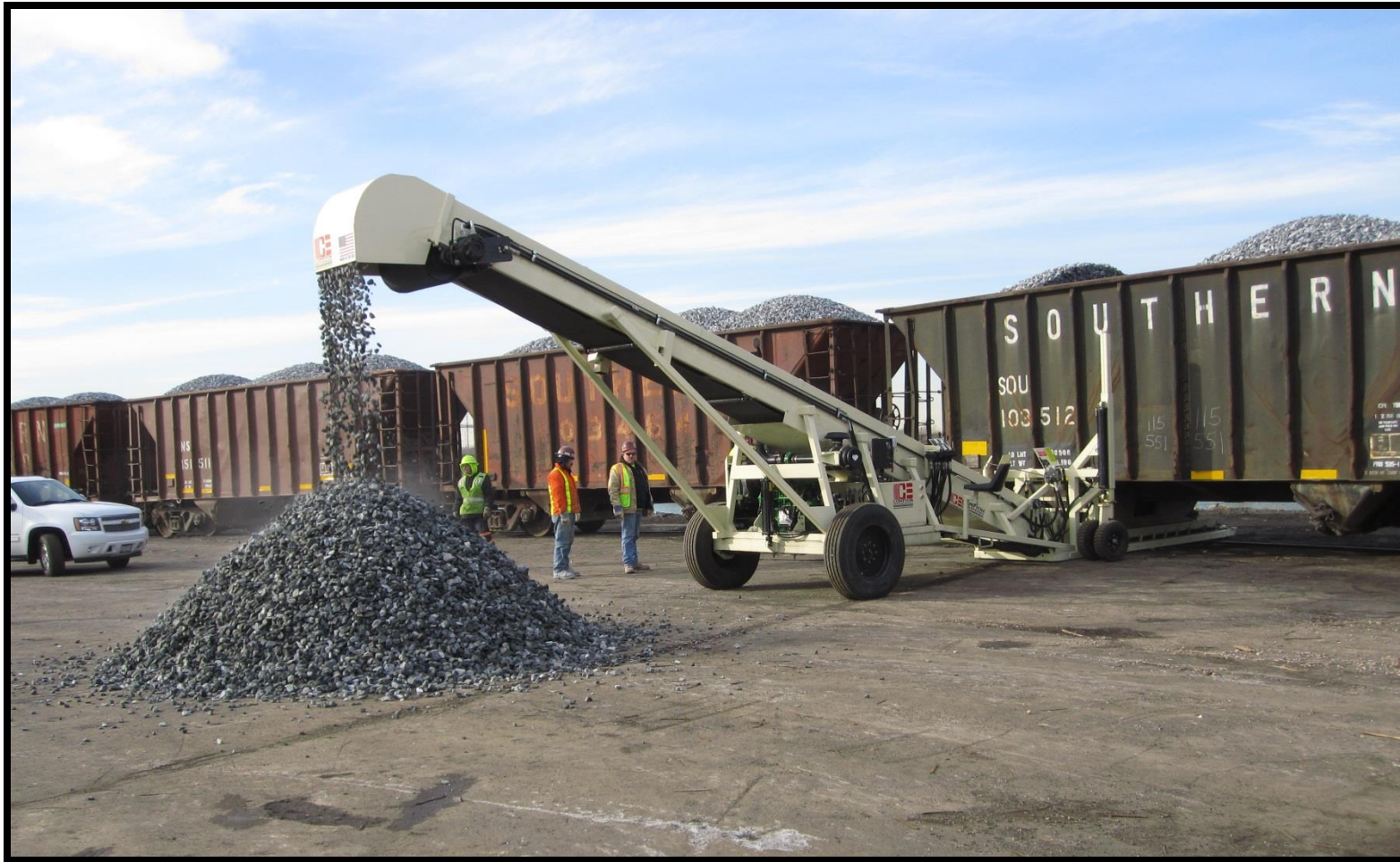
Unloading of granite ballast from rail cars
