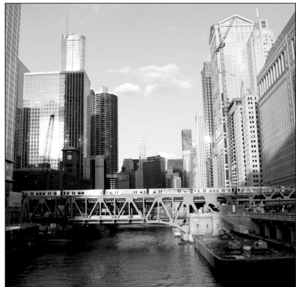
By coordinating critical CTA track work at the Tower 18 junction with CDOT's reconstruction of the 90-year old Wells Street Bridge, both agencies achieved cost savings and reduced the work's impact on the roughly 40,000 CTA rail customers who travel across the bridge each weekday.
