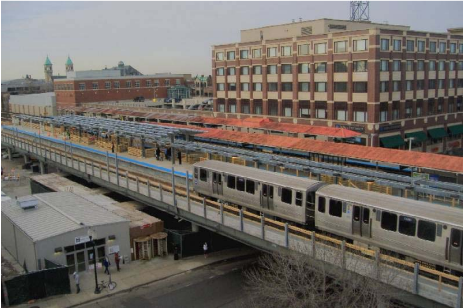
New track 4 and platform at Fullerton
