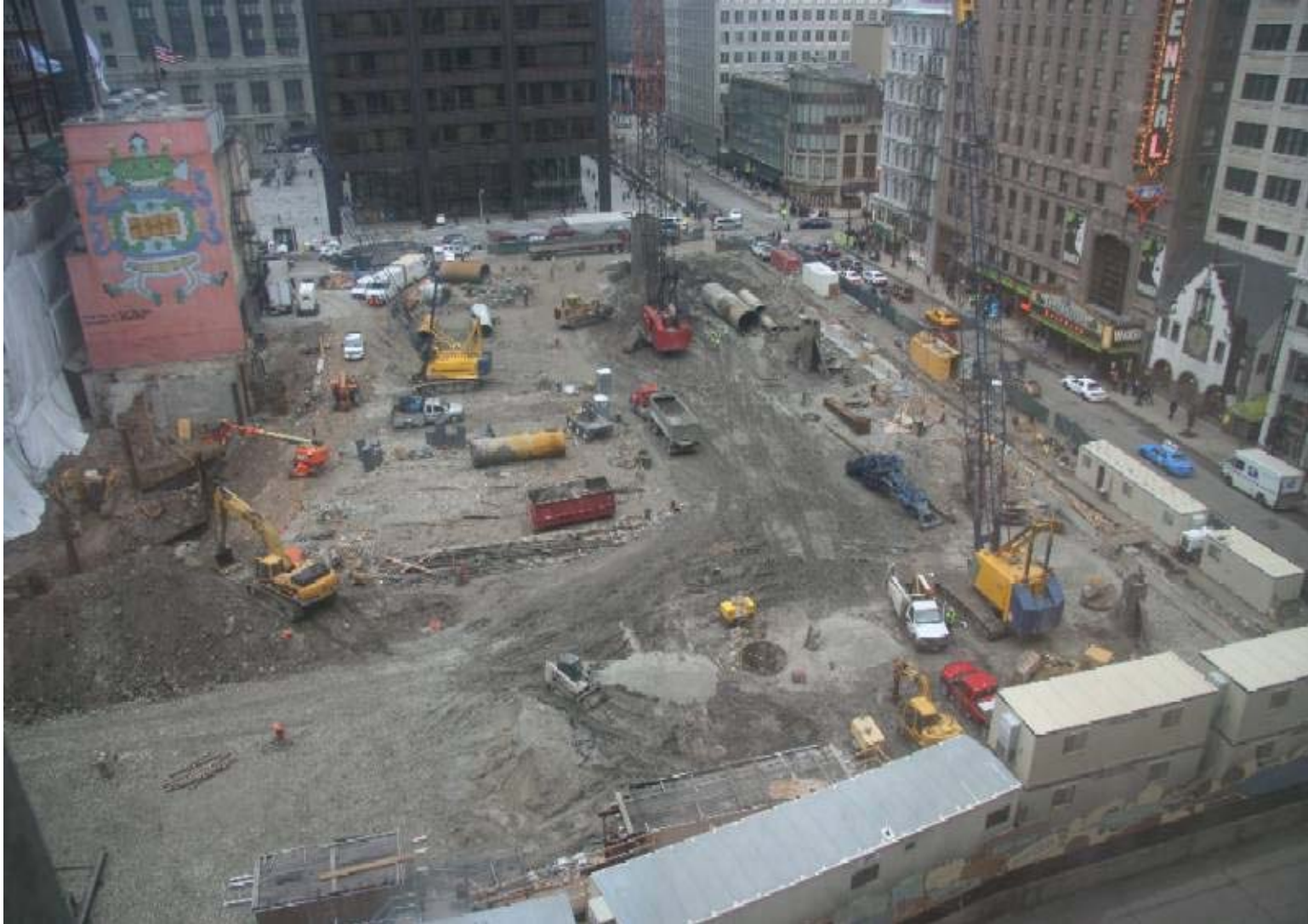
Block 37 work site looking south
