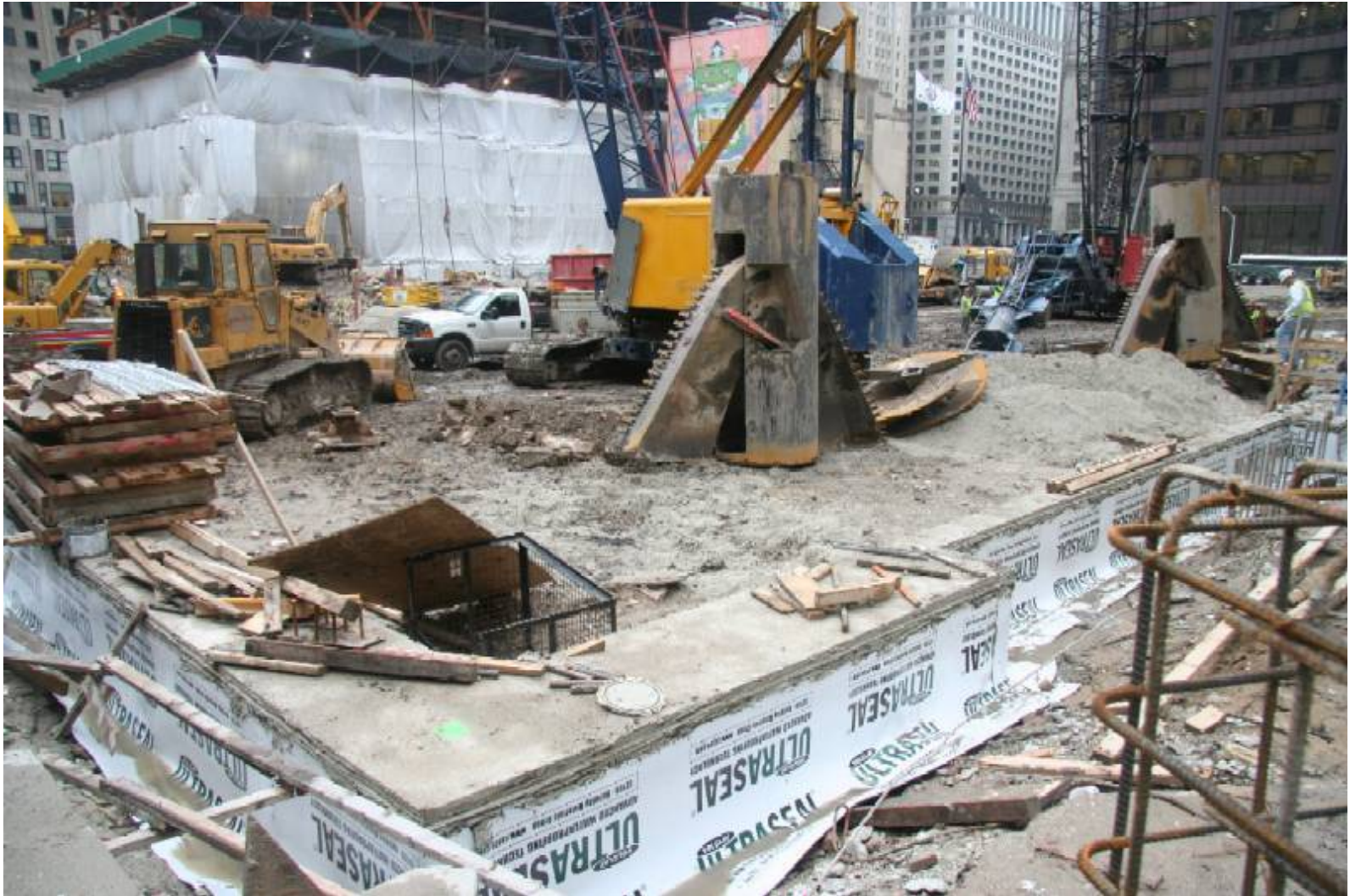
Completion of slurry wall at corner of State/Randolph
