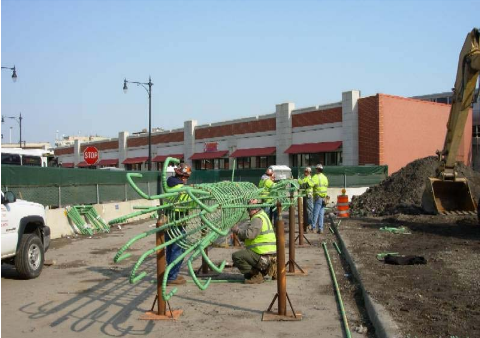
Construction of caisson reinforcing steel cages
