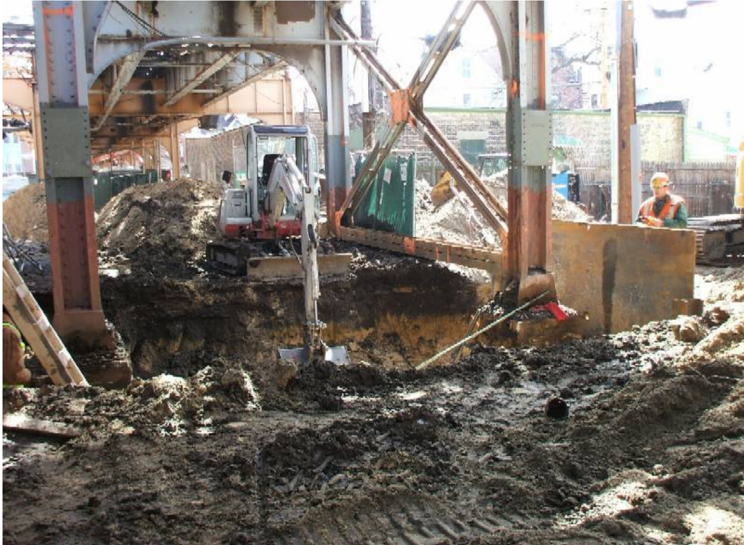
Addison Station foundation replacement
