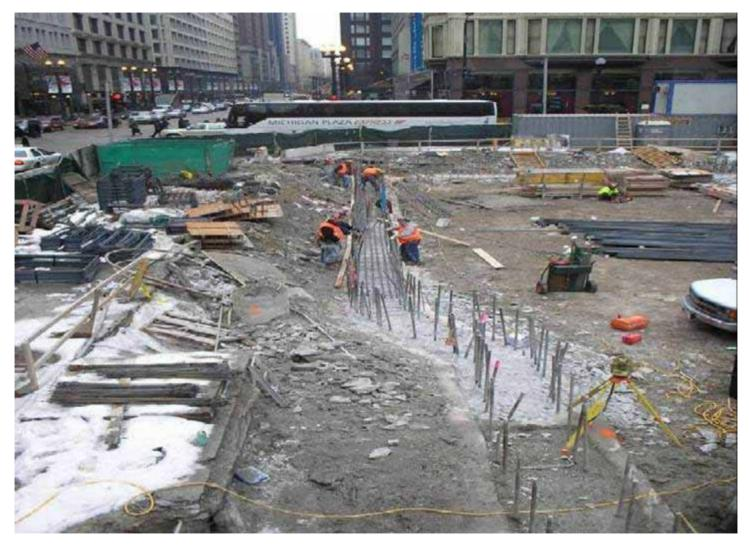
Constructing rebar cages for slurry wall cap beam
