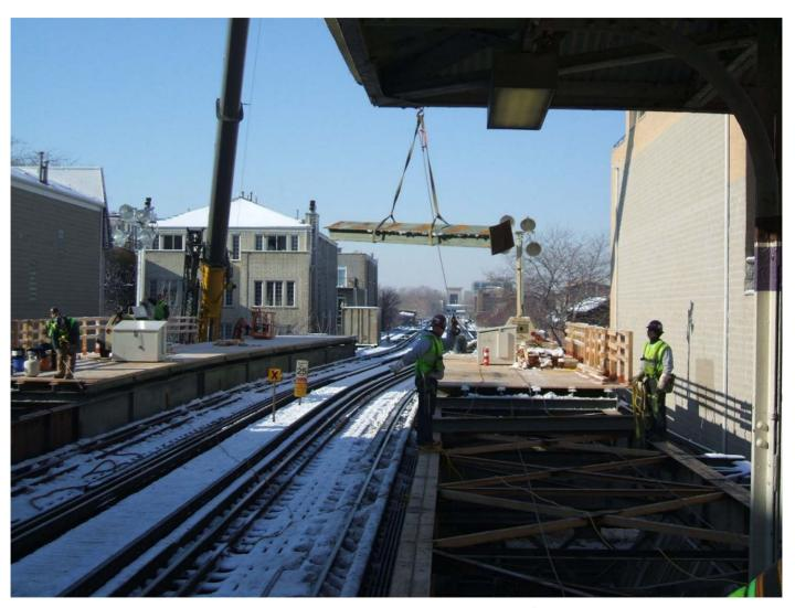
Installation of new platform steel at Sedgwick
