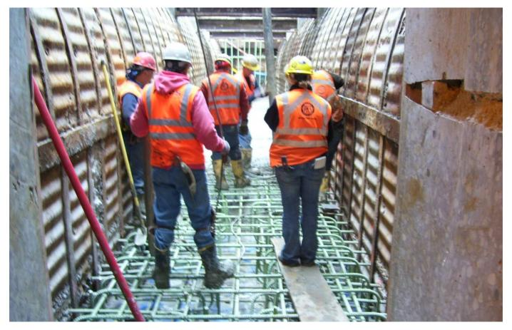
Concrete floor slab pour between subway tunnels for Chestnut Relay room
