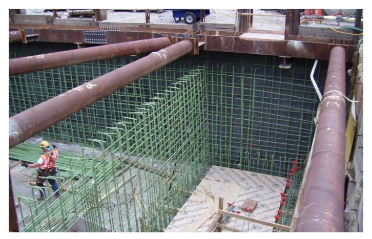
Rebar installation for Belmont Relay Room
