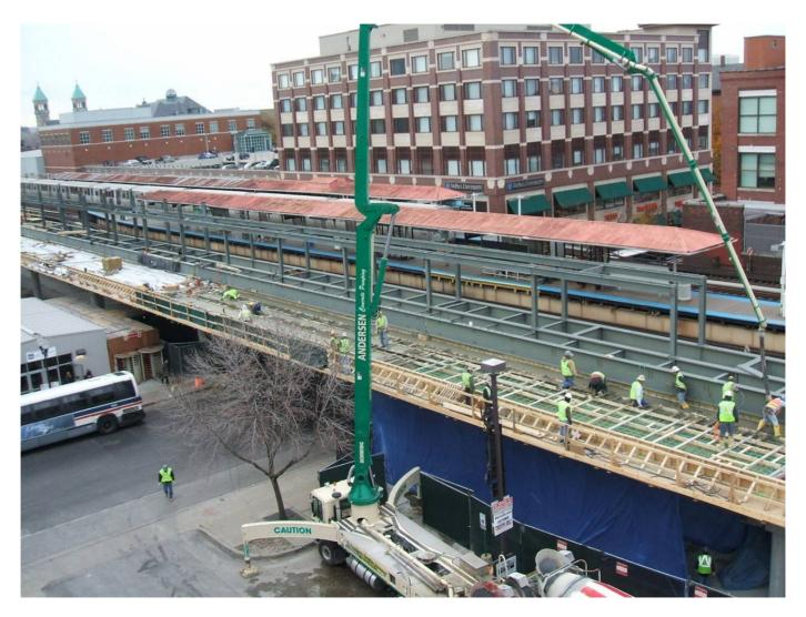
Pouring new concrete track bed at Fullerton
