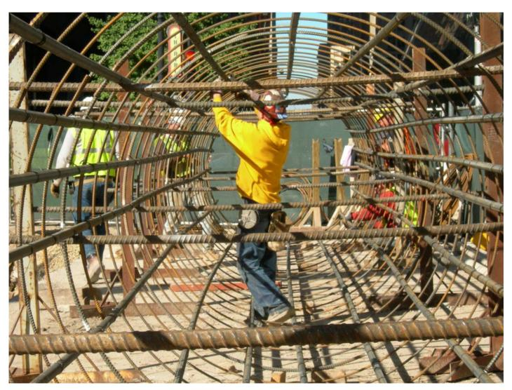
Assembling of caisson rebar frames
