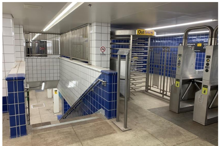
Photos of the Division Blue Line station before and after station improvement work was performed as part of the Your New Blue program.
