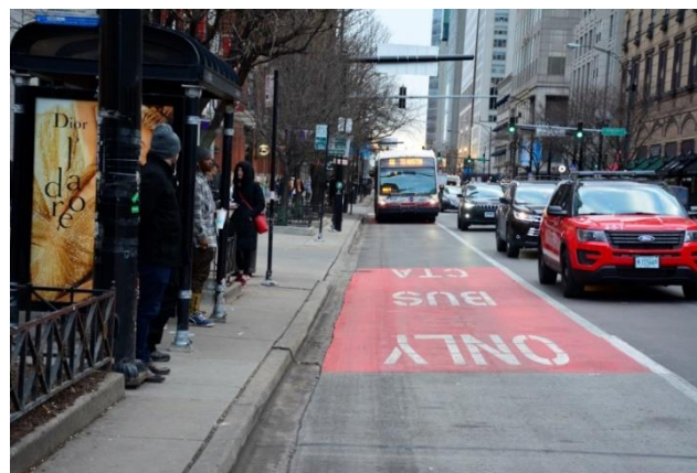
A new bus-only lane installed along a portion of Chicago Avenue as part of the Bus Priority Zone program to help improve service reliability along the #66 Chicago route.
