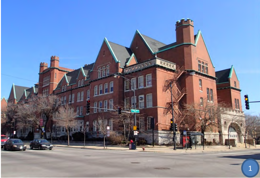
4015 North Ashland Avenue
