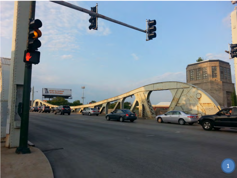
North Ashland Avenue Bridge
