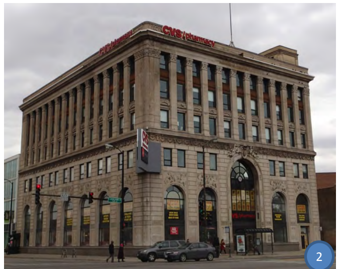
1200 North Ashland Avenue
