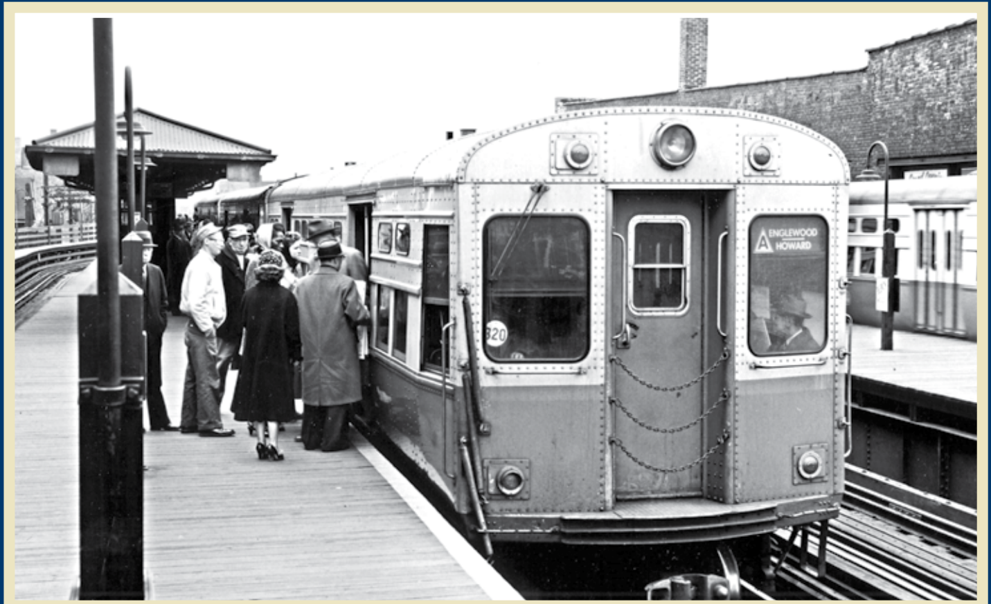
It's the early 1960's, and customers are boarding a southbound 6000-series train at the Belmont station on the North-South through-route. These cars were part of a fleet of 720 6000-series cars CTA purchased as part of their efforts to modernize the 'L' fleet. These cars were the mainstays of the North-South Route (Howard-Englewood-Jackson Park) for decades.
